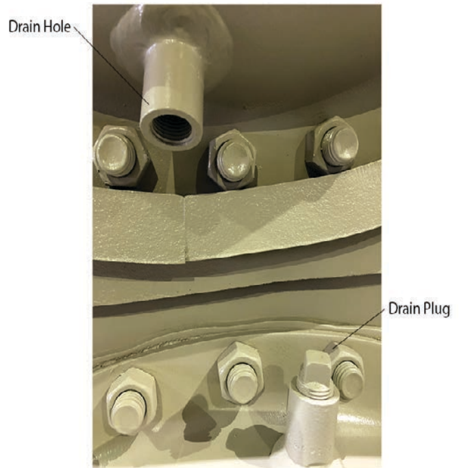
Figure 15: Drain Plug Installation
