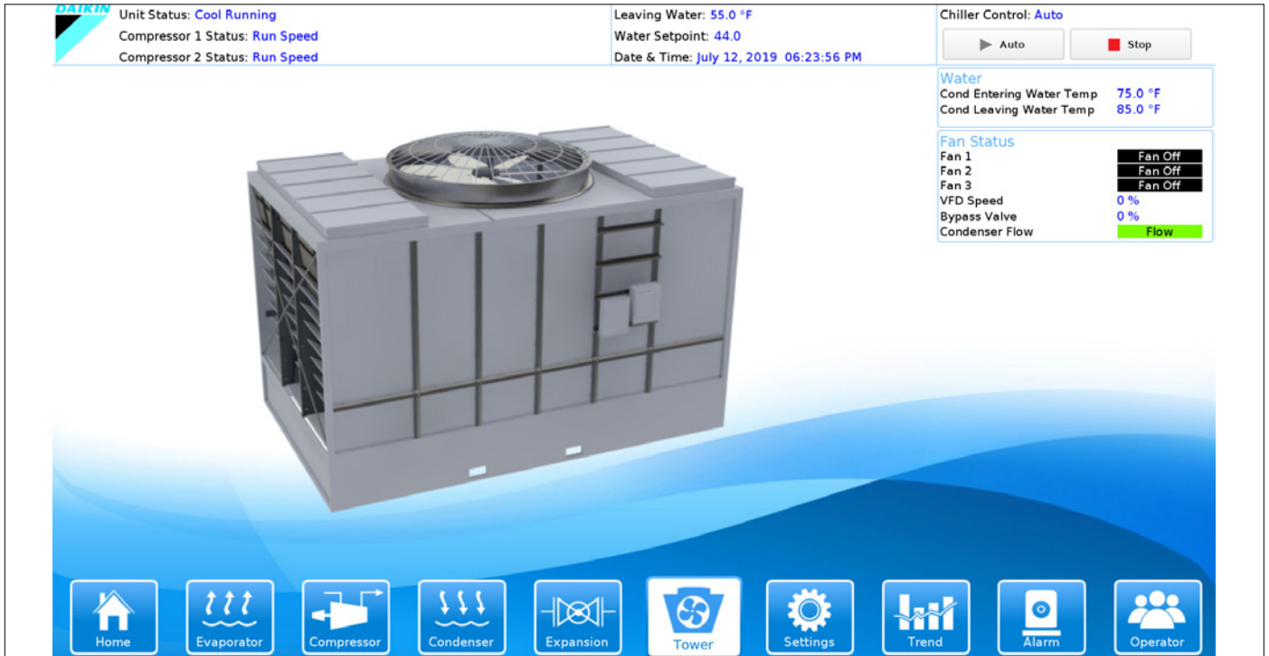
Figure 38: Cooling Tower Information
