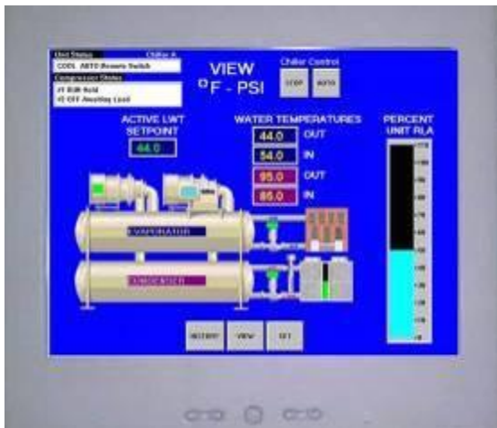
Figure 42, MicroTech II Control Panel
