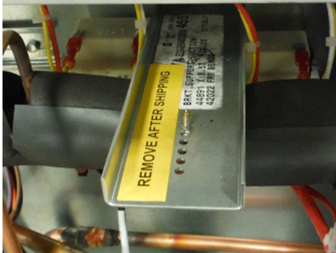
Figure 20: Compressor Brackets
