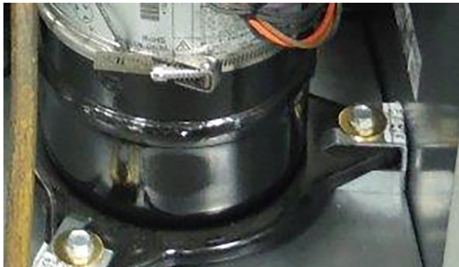
Figure 20: Compressor Brackets
