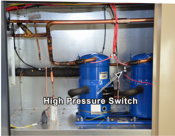
Figure 35: High Pressure Switch
