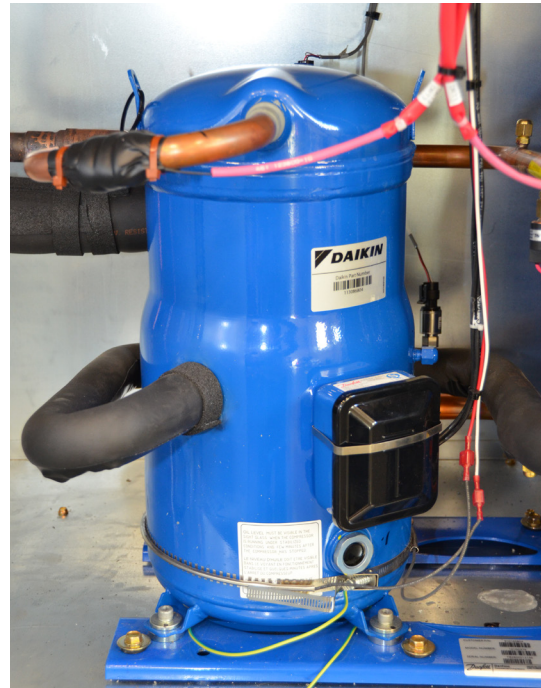
Figure 34: Compressor Suction and Discharge on DPS 025–028 units
