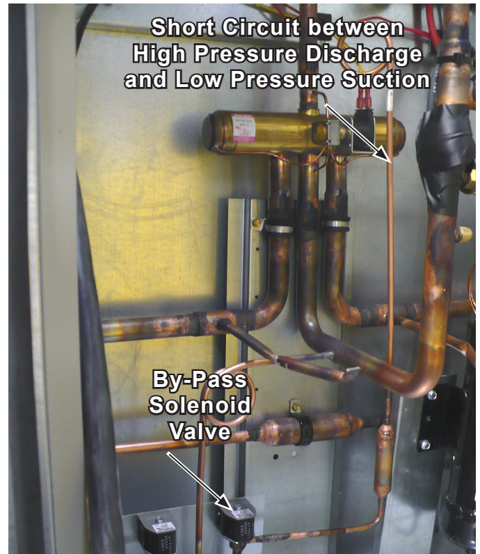
Figure 30: By-pass Solenoid Valve
