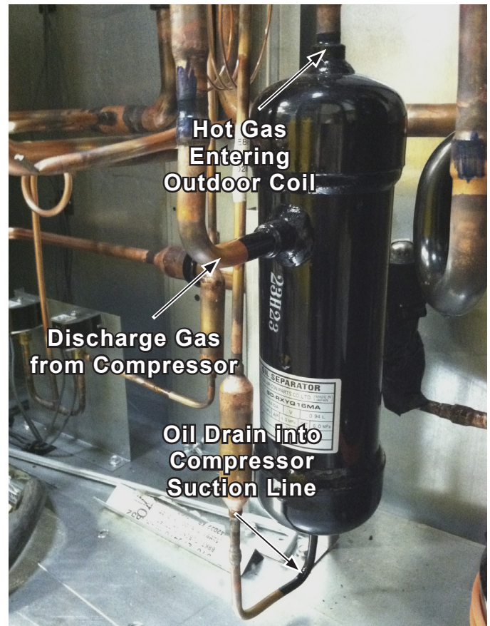
Figure 24: Oil Separator
