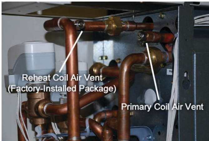
Figure 18: Coil Air Vents
