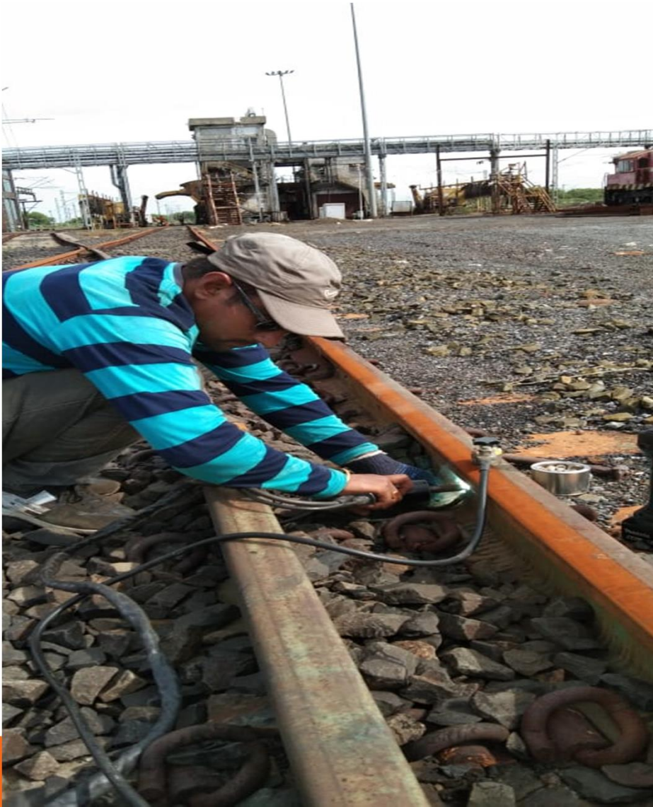
CONTINUITY BOND INSTALLED ON TOUNGE RAIL AT NTPC MAUDA, NAGPUR YEAR 2017 A/C RITES LTD
