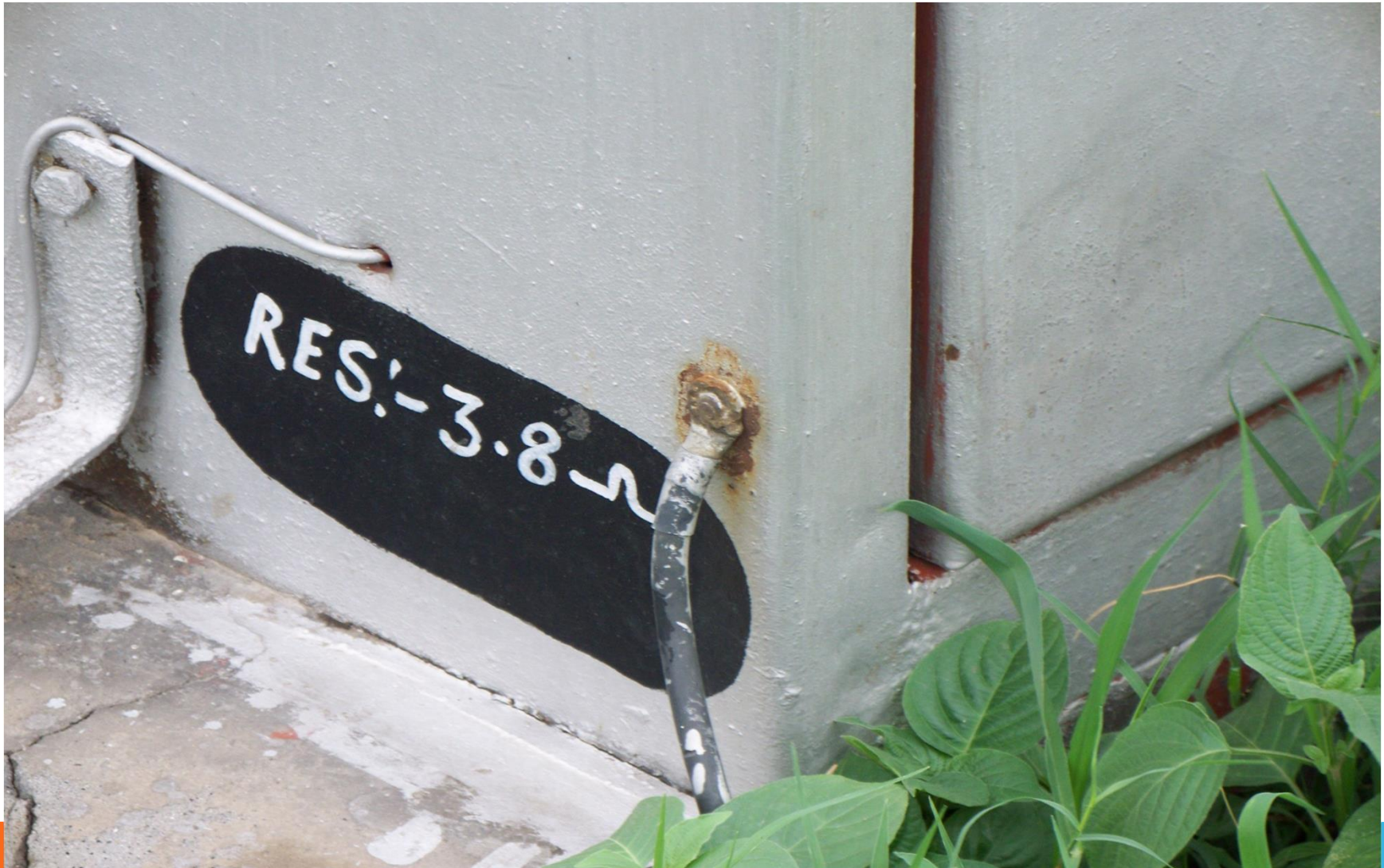
PIN BRAZED CONNECTION ON LOCATION BOX AT VIVEK VIHAR, DELHI IN YEAR 2015
