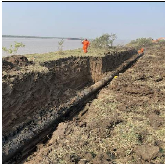
RIVERSIDE PIPE IN TRENCH
