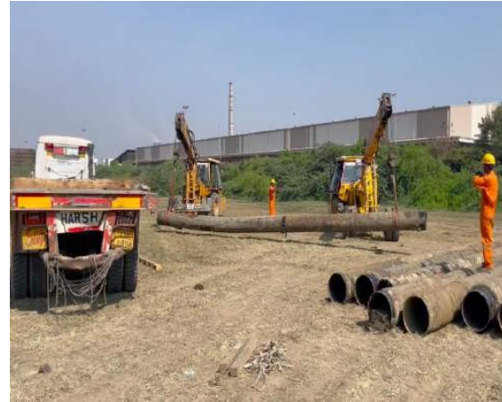
PIPE LIFTING BY HYDRA
