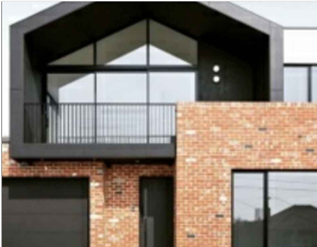
A FEATURED BRICKWORK
