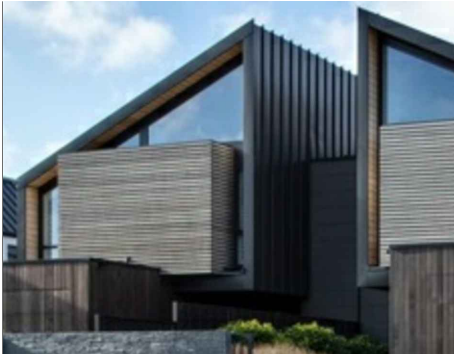
B COLORBOND WRAPPING ROOF SHEETING + WALL CLADDING
