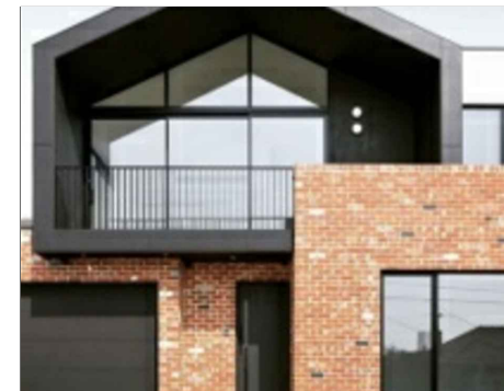
A FEATURED BRICKWORK
