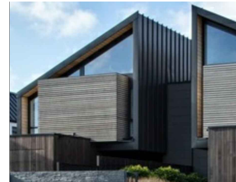
B COLORBOND WRAPPING ROOF SHEETING + WALL CLADDING
