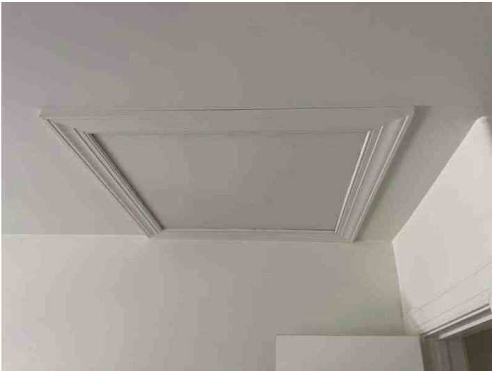
Bedroom -attic entrance, access to heater
