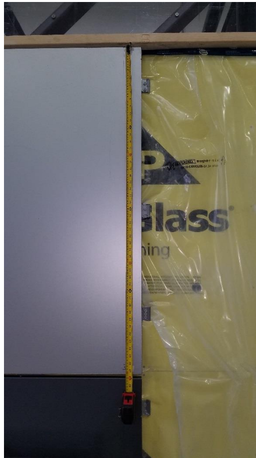
Photo No. 2 Clip Spacing for the Panels
