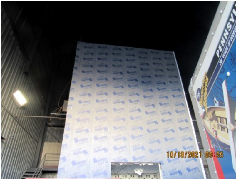
Photo No. 1 Weather barrier installed
