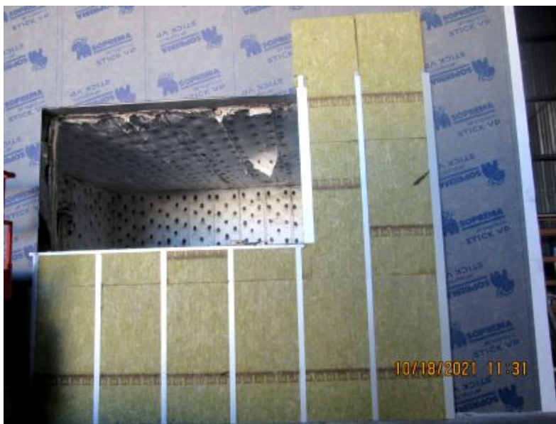
Photo No. 2 Installation of insulation
