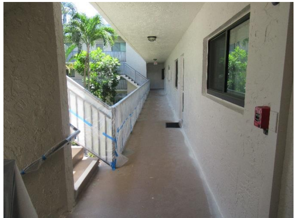
View of typical breezeway.
