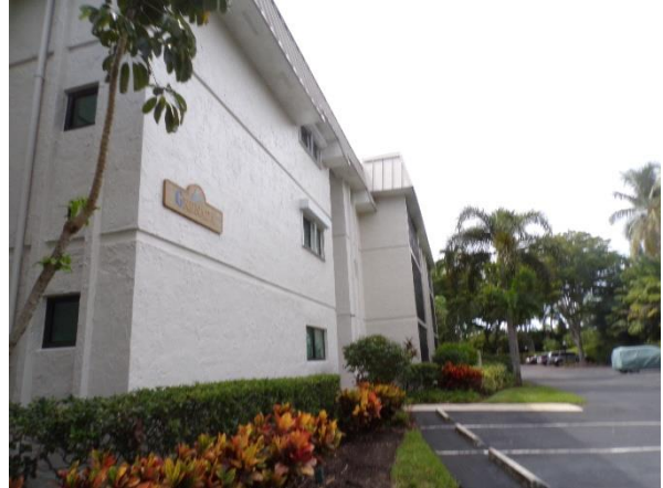
View of west elevation.
