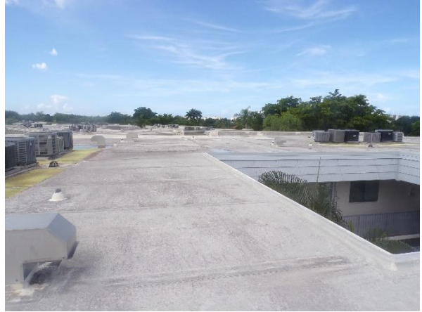
Overall view of single-ply roof.
