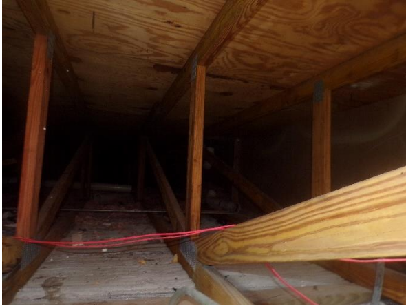
Partial View of attic.
