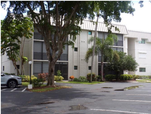
View of south elevation.
