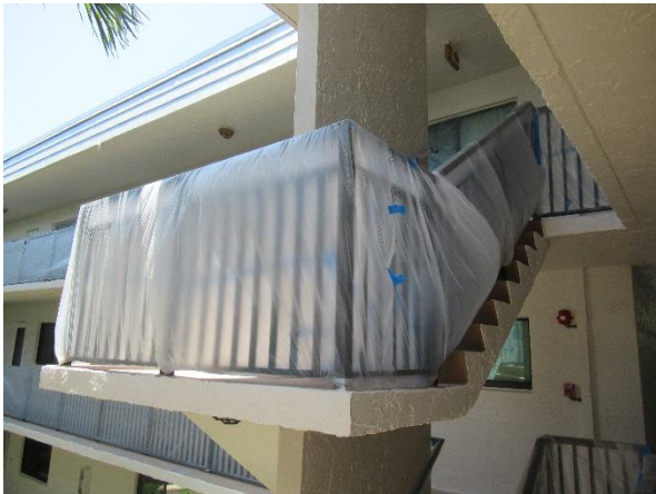
Overall view of 1 st floor walkway.
