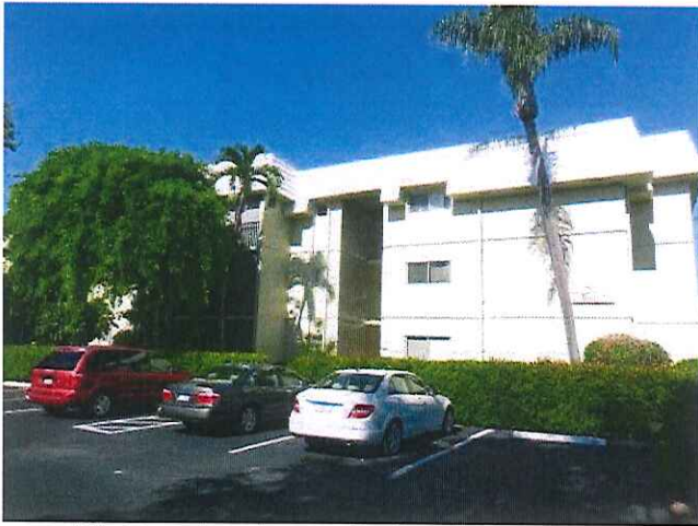
#1 Front view of the building
