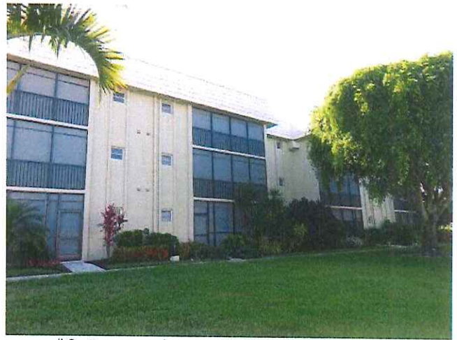
#2 Rear view of the building
