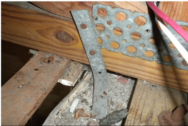
Roof to Wall Attachment
