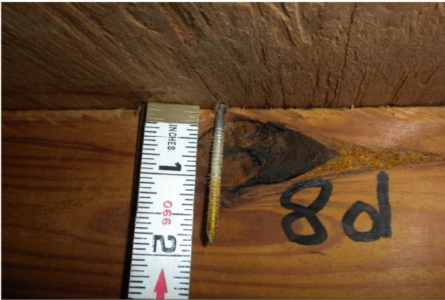
Roof Deck Attachment
