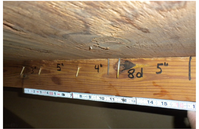
Roof Deck Attachment
