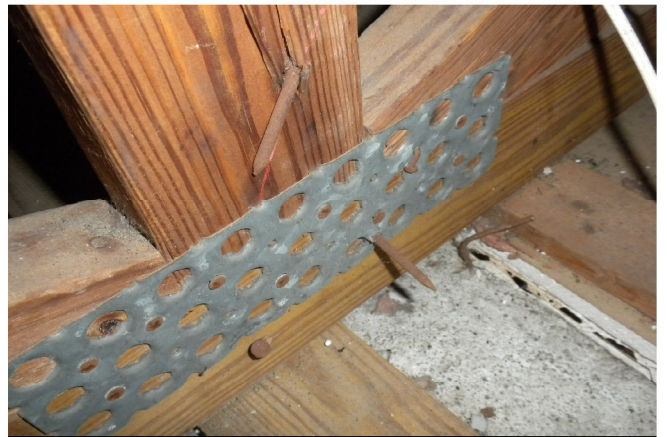
Roof to Wall Attachment
