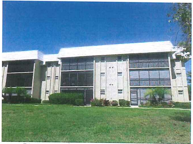
#2 Rear view of the building
