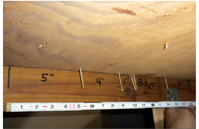
Roof Deck Attachment
