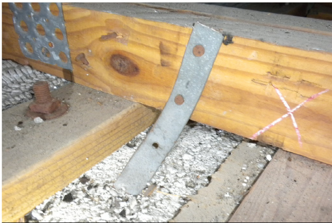
Roof to Wall Attachment
