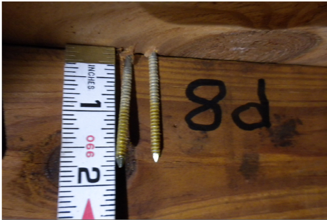
Roof Deck Attachment
