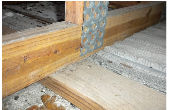
Roof to Wall Attachment
