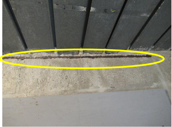
View of exposed rebar on wall of 1 st floor electrical room.
