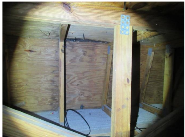
View of water staining on attic sheathing.
