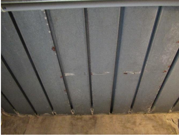
View of rust staining on steel deck on ceiling of 1 st floor electrical room.
