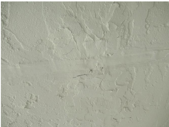
View of stucco crack on breezeway.
