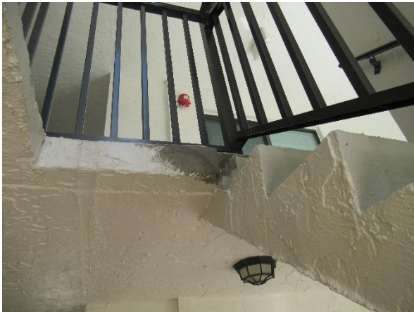
View of previous concrete repair.
