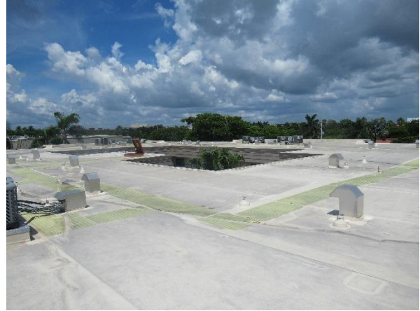
Partial view of TPO roof.
