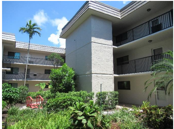
Overall view of courtyard.
