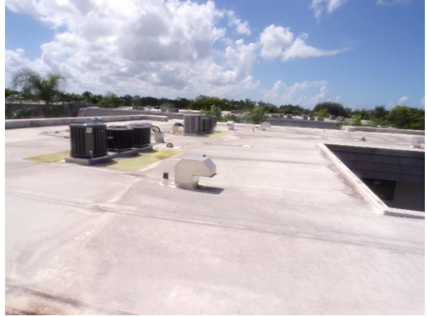
Overall view of single-ply roof.
