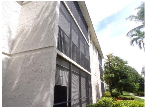
Partial view of east elevation.
