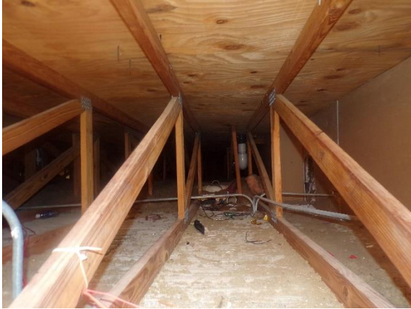
Partial View of attic.
