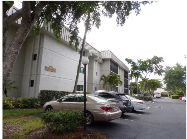
View of west elevation.
