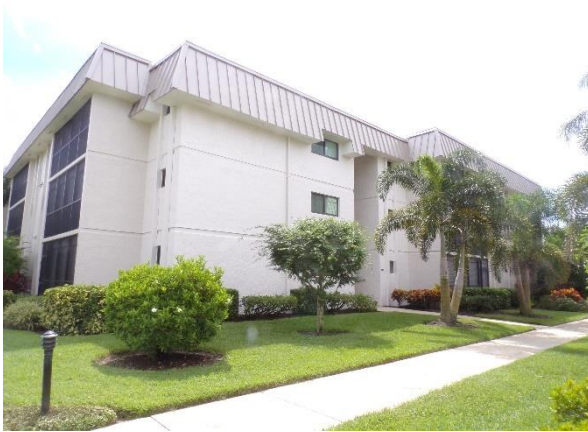
View of north elevation.
