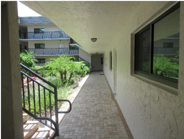
Overall view of 1 st floor walkway.
