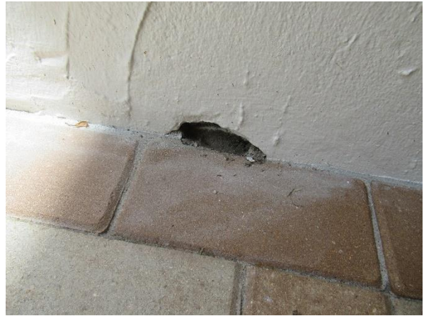
View of delaminated stucco on wall of 1st floor breezeway.
