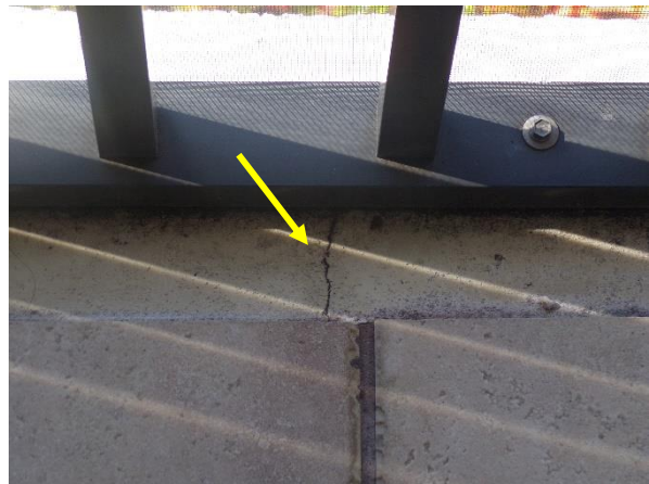
Typical hairline crack on slab edge, lanai of unit 28.
