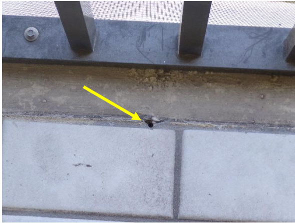
View of unsealed penetration in lanai of unit 33.
