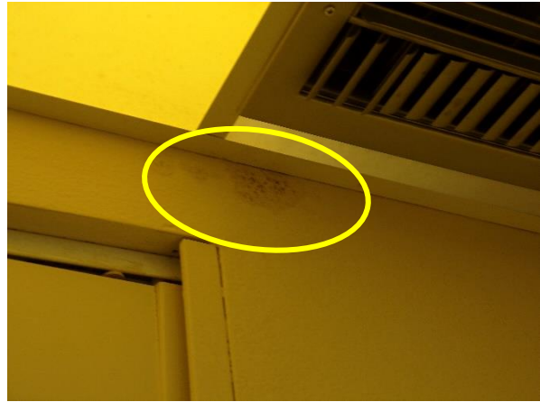
View of possible water intrusion in unit 31.
