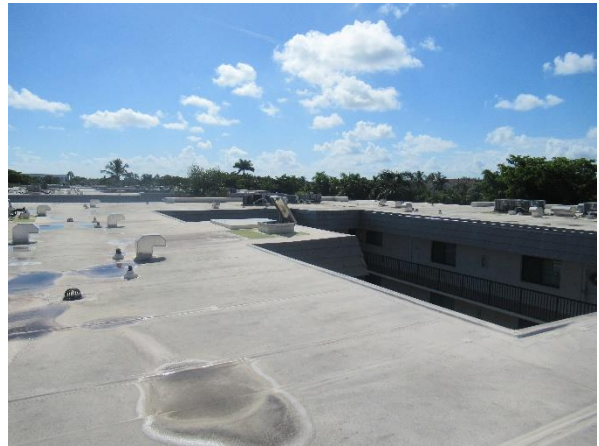
Overall view of TPO roof.
