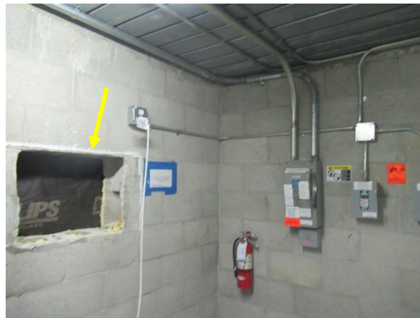
View of missing section of CMU wall.
