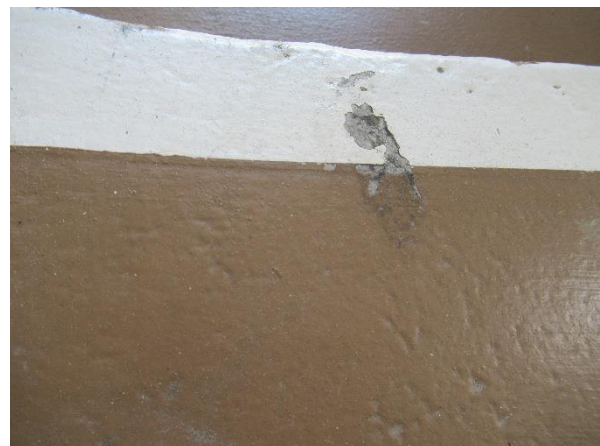
View of typical chipped coating on stairs.
