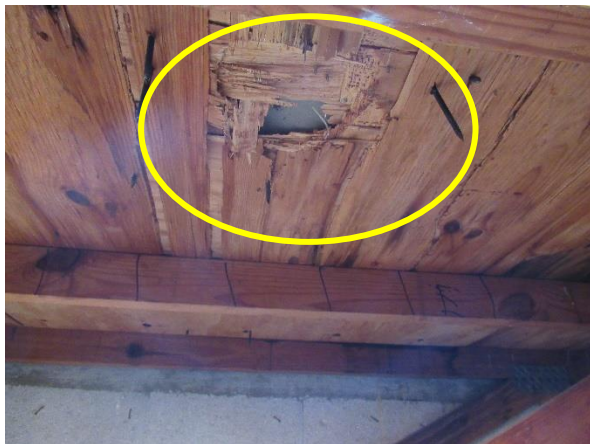
View of damaged roof sheathing.
