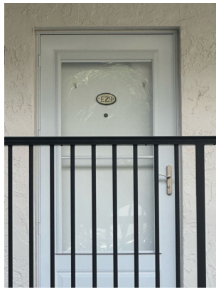
Unprotected Opening
