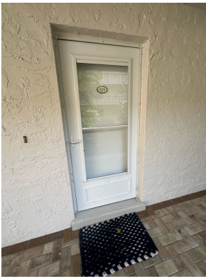
Unprotected Opening
