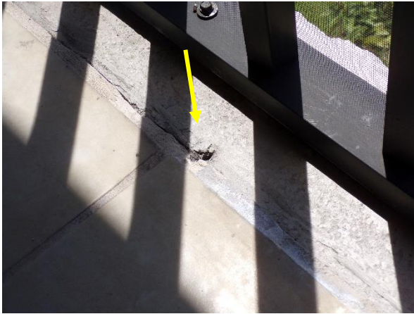
View of unsealed penetration in lanai, unit 37.
