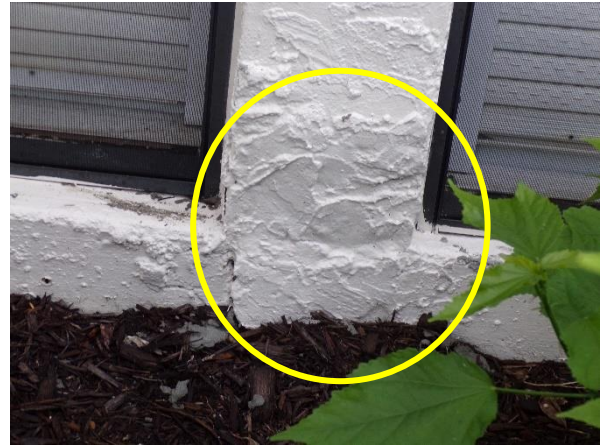
View of delaminated stucco on exterior wall.
