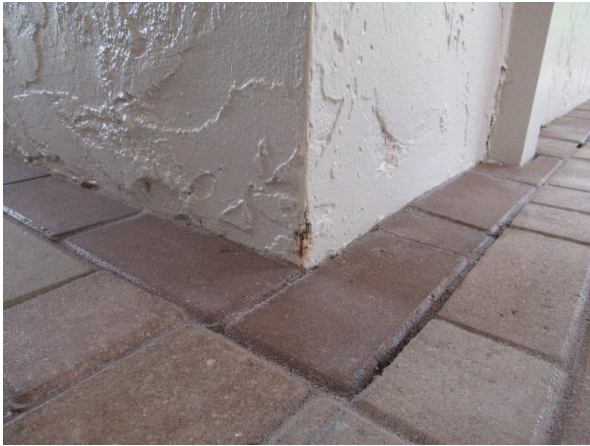
View of rust staining on breezeway of 1st floor.
