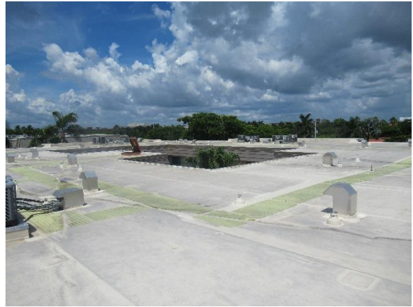
Overall view of TPO roof.
