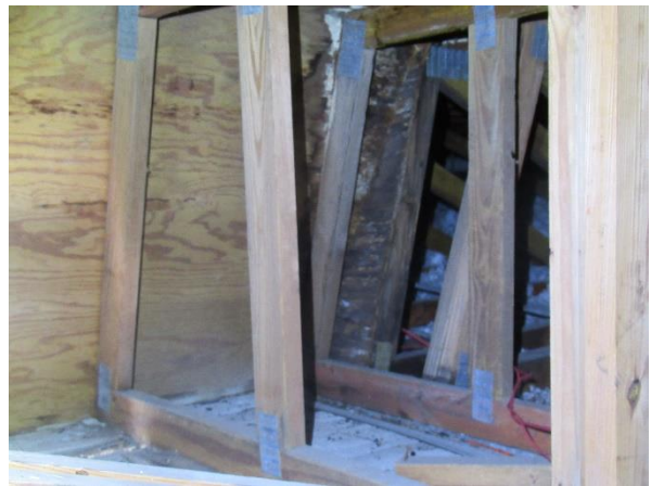
View of water staining in attic.
