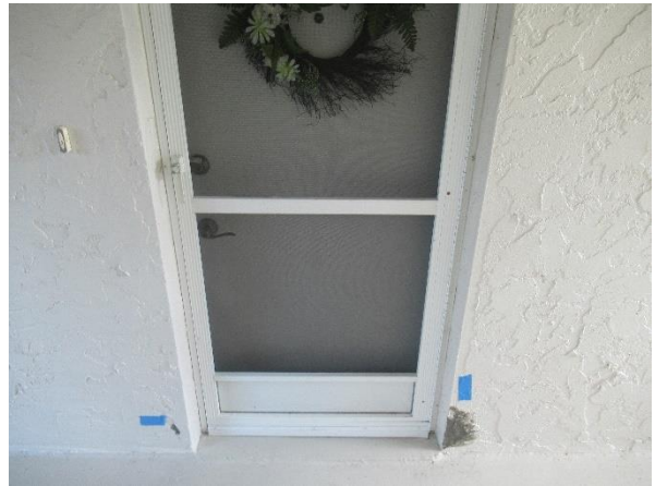
View of previous stucco repairs.
