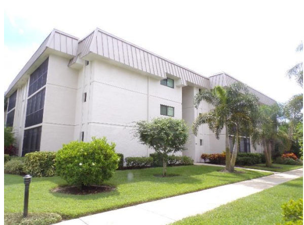
View of west elevation.
