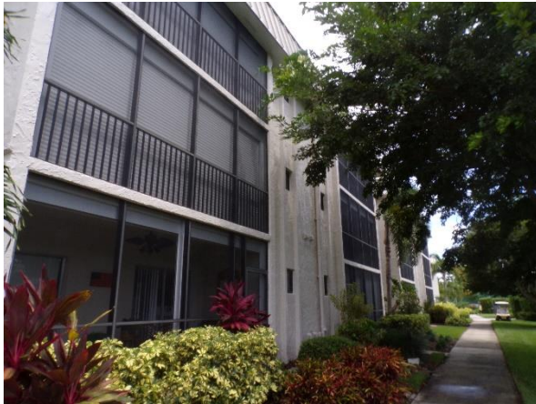
View of north elevation.
