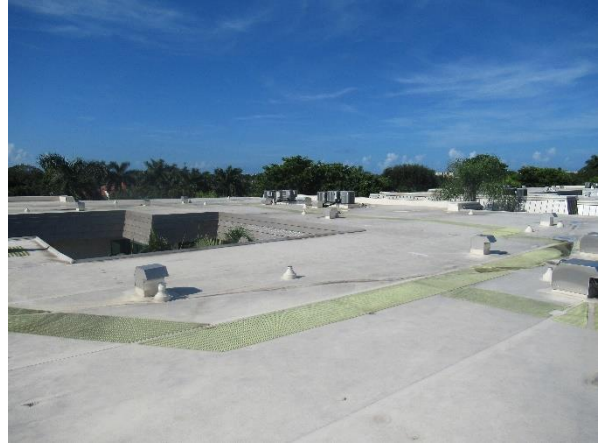
Overall view of single-ply roof.
