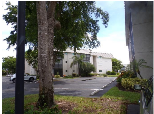
Partial view of east elevation.
