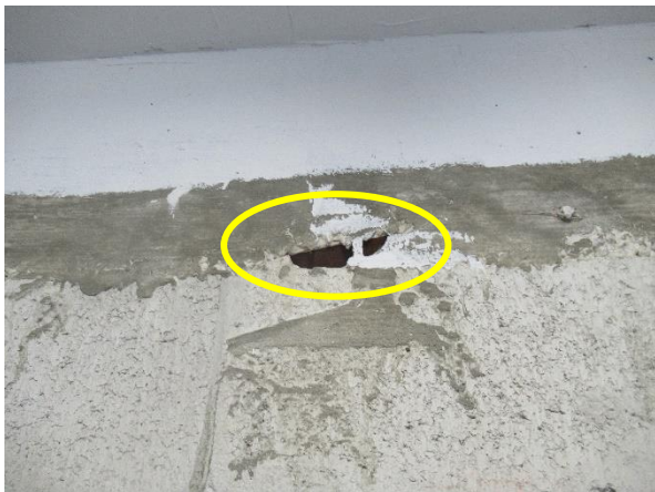
View of exposed rebar in 3 rd floor mechanical room.
