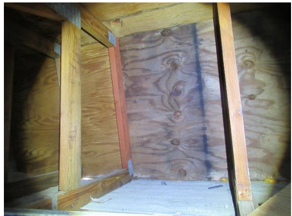
View of water staining on roof sheathing.
