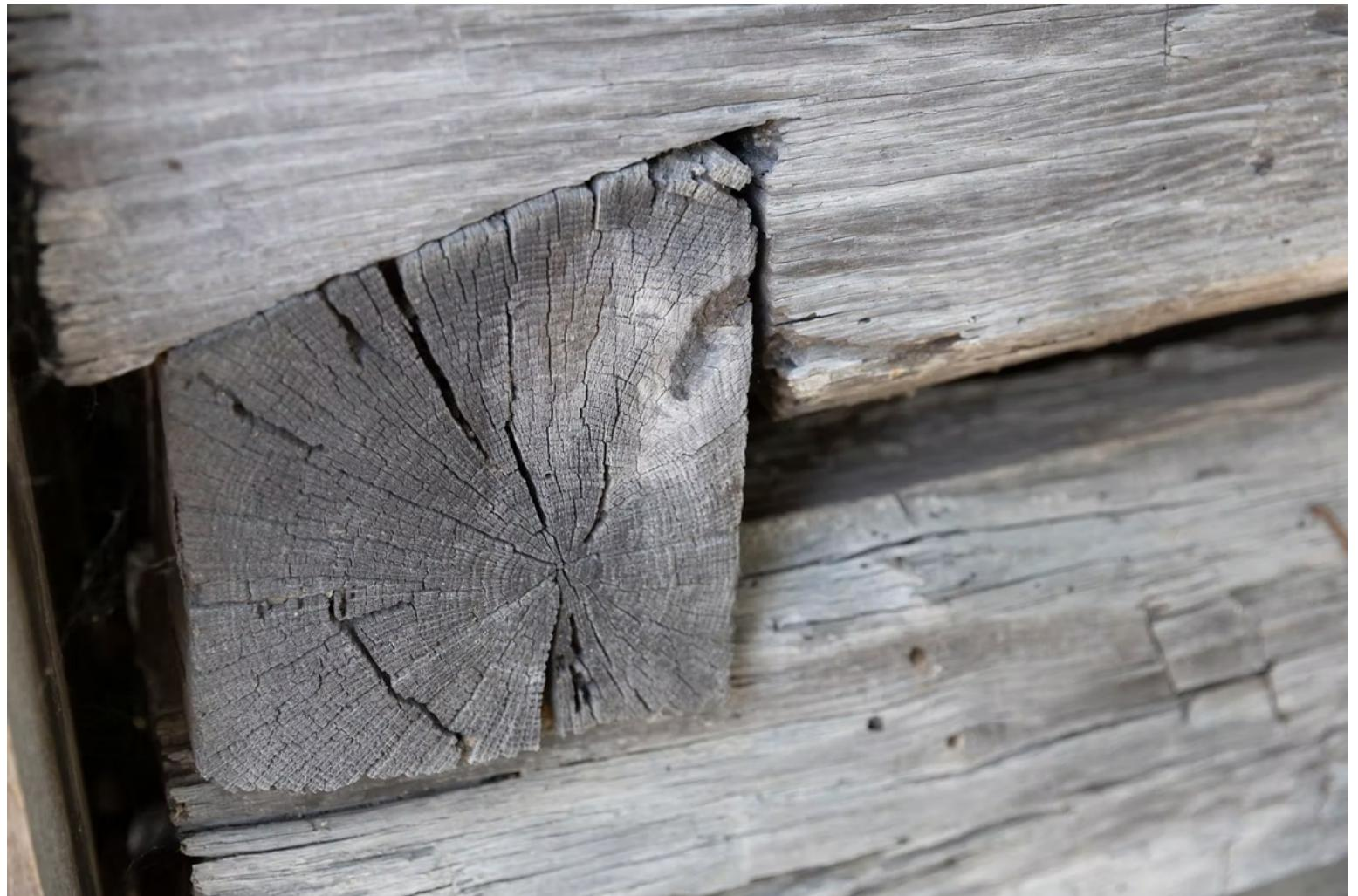
Dovetail joints make it able to withstand centuries without even a single nail to hold it together.
