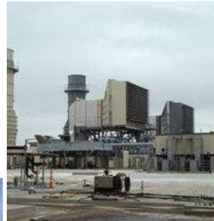
Xcel Energy's Jones Station, TX.
