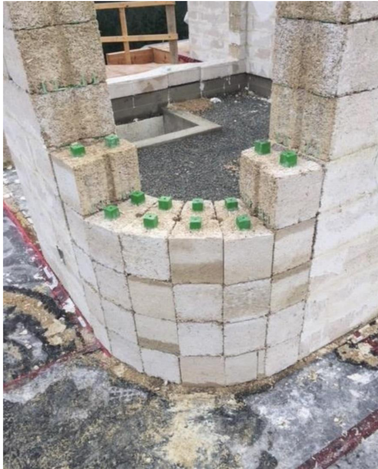
Figure 8 • Capability of hempcrete for curved wall to enhance esthetic appeal. Reproduced with permission from Keinonen [39].
