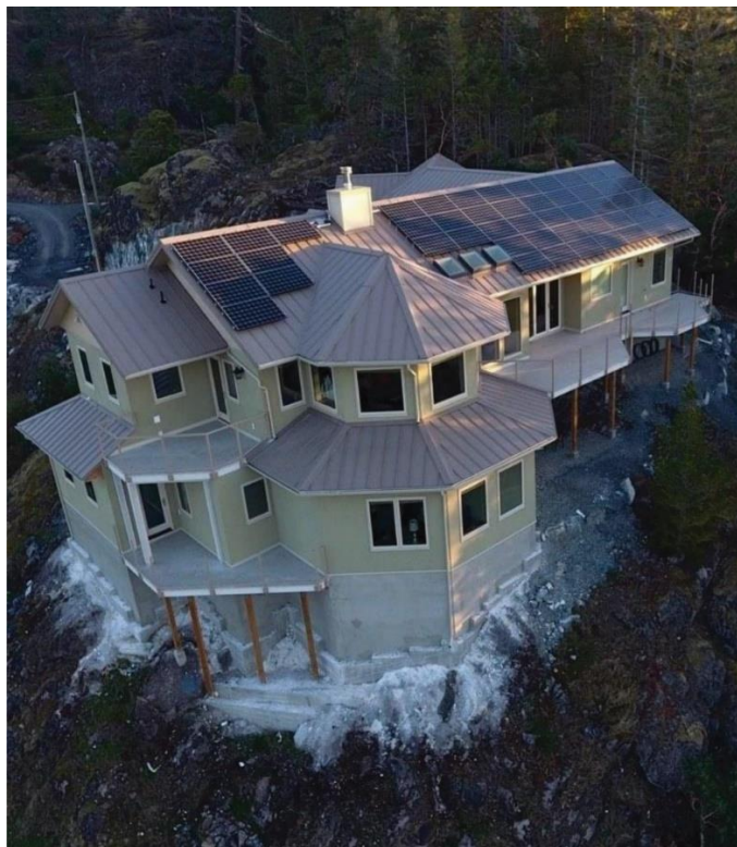
Figure 7 • Serial view of the Harmless Home, a hempcrete-built residence in British Columbia, Canada. Reproduced with permission from Keinonen [39].
