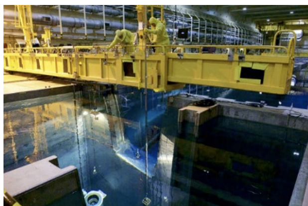
Idaho Nuclear Technology and Engineering Center workers transfer Experimental Breeder Reactor-II SNF from the Chemical Processing Plant-666 basin to a shipping cask.
