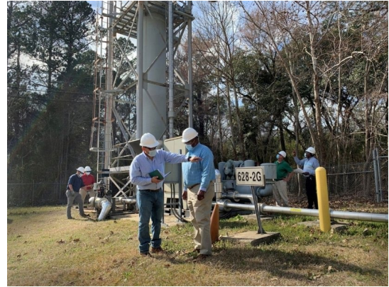
A Savannah River Site project team inspects a pump-and-treat groundwater treatment system.
