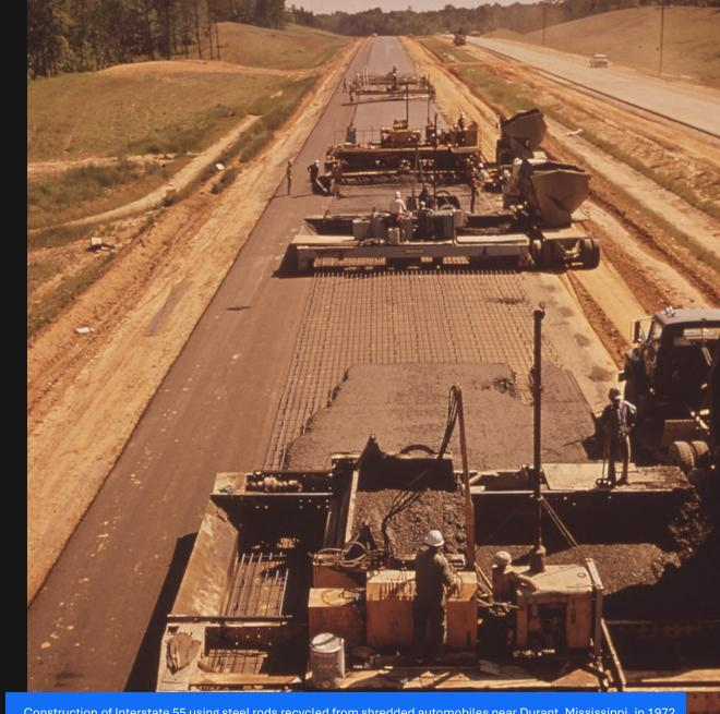
state 55 using steel rods recycled from shredded automobiles near Durant, Mississippi, in 1972
