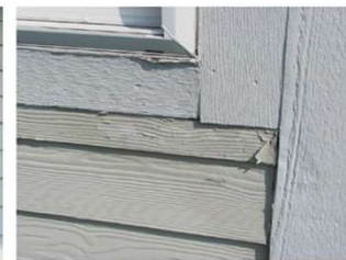
Peeling paint finish at Unit 300
