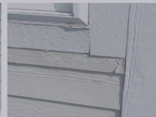
Peeling paint finish at Unit 300
