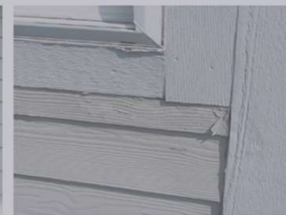
Peeling paint finish at Unit 300
