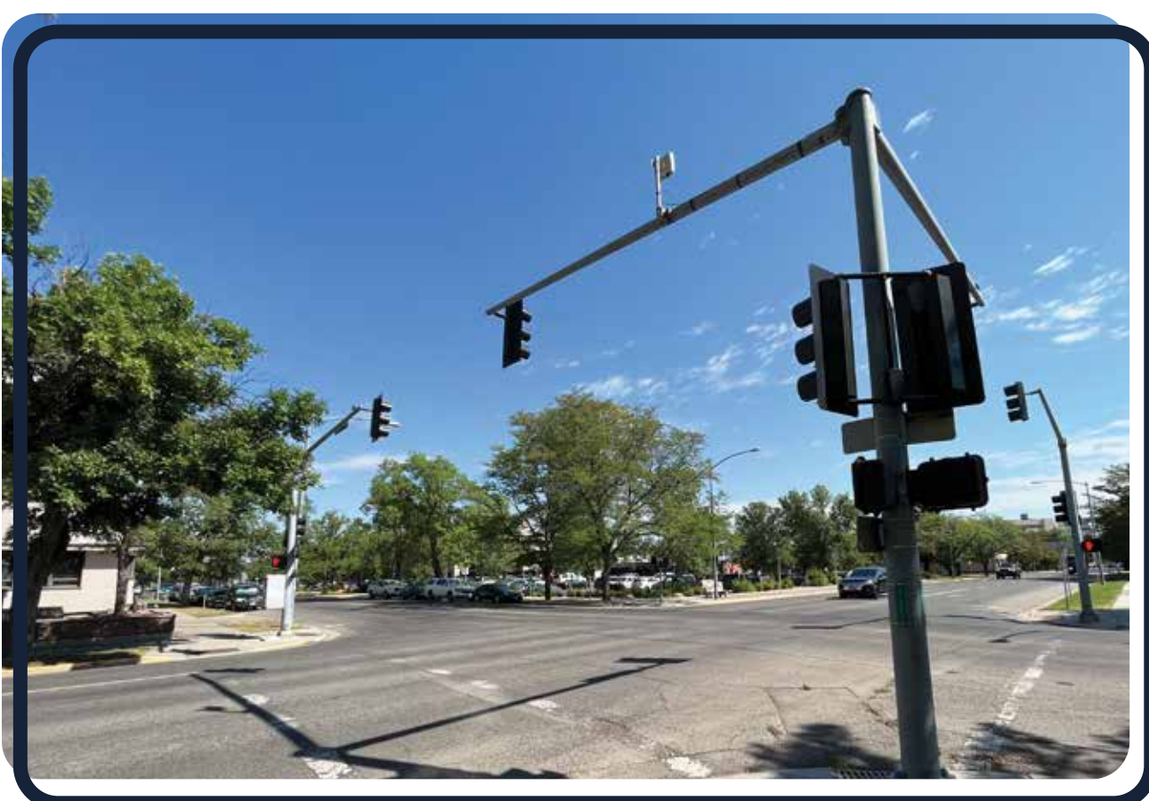
Traffic signals will be removed and replaced with stop-control devices at North 32nd Street and 3rd Avenue North and North 32nd Street and 2nd Avenue North.
