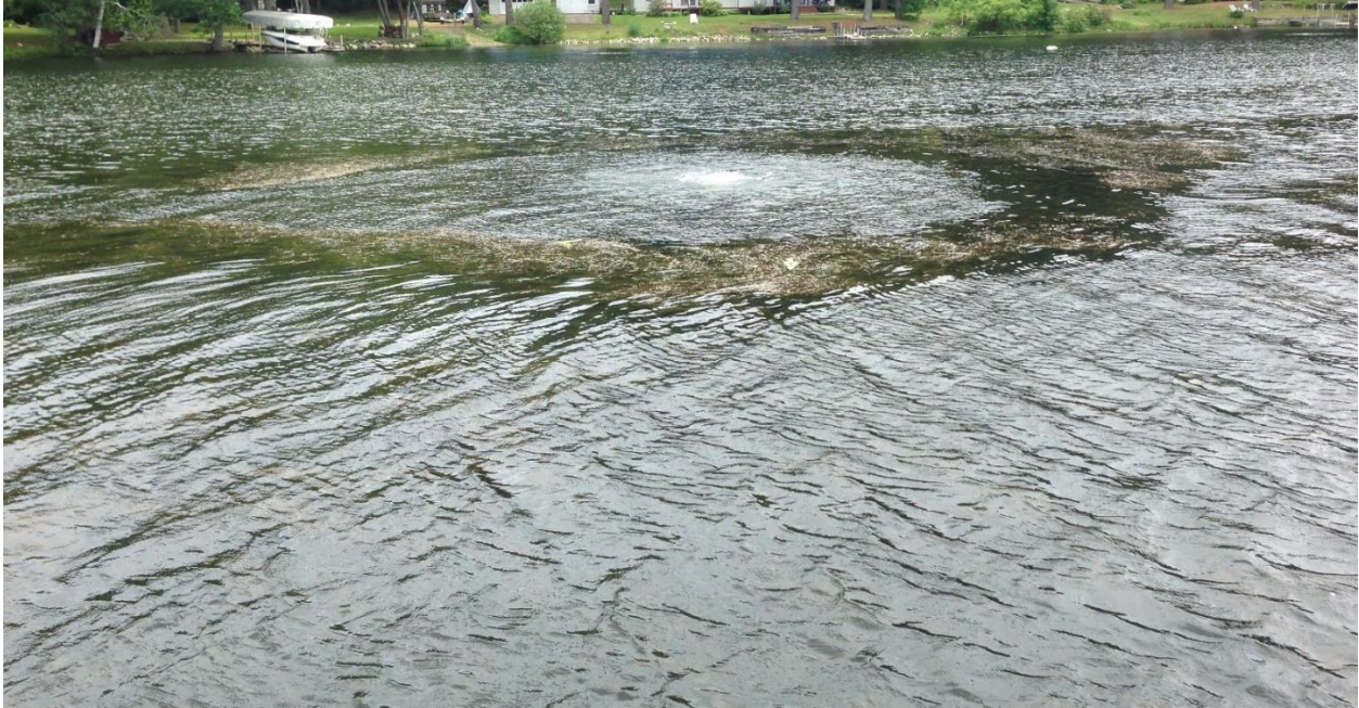
Compressed air diffuser installed in Little Lake St. Catherine, Wells (Photo Credit VT DEC)
