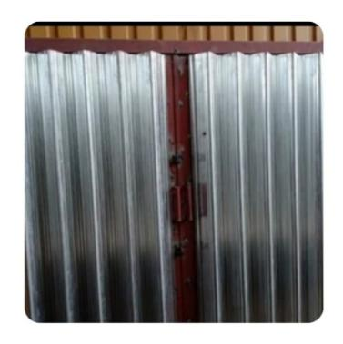
A sliding shutter is a type of window covering that operates by sliding horizontally along a track, usually mounted on the exterior of a building, allowing users to open or close the shutter panels to control sunlight, privacy, and ventilation by moving them sideways to cover or reveal a window opening.
