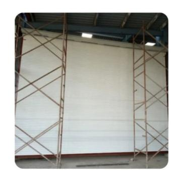
An automatic rolling shutter is a type of door or window shutter made up of horizontal slats that can be rolled up or down to open and close an, operated by a motorized mechanism that can be controlled remotely or via a wall switch
