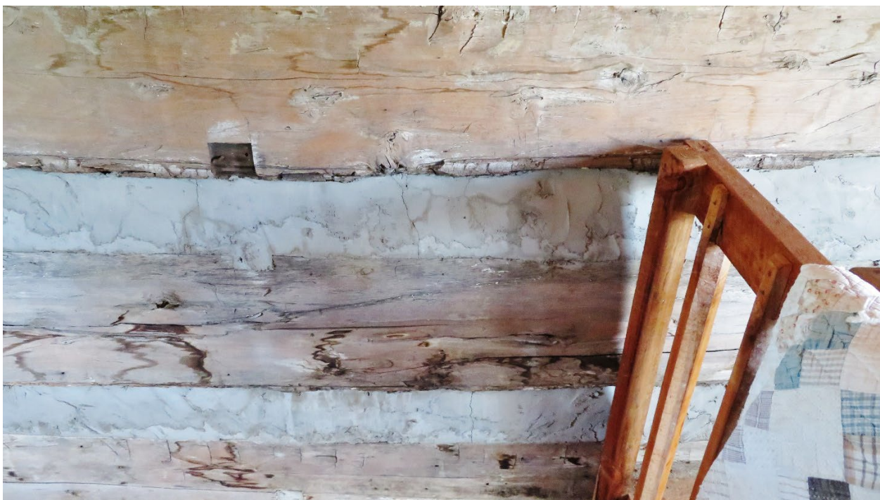
Fig. 6. A mortise in the wall indicates the position of the original railing at the stairwell opening. There is another mortise for the header directly below. The new railing position (right) takes away floor space on the second level.
