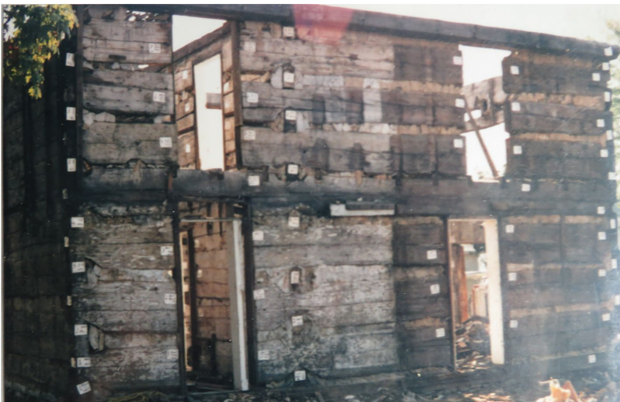
Fig. 4. This is a rear view of the log home before it was disassembled in 1986. The doorway on the left had been re-framed at some time in the past, but the height of the rough opening indicates that it was originally cut for a door. The bottom was filled in two logs higher during re-modeling, making it a window. The opening on the lower right, which is relatively lower at the top, is now used for a door, but its height indicates it was originally a window.
