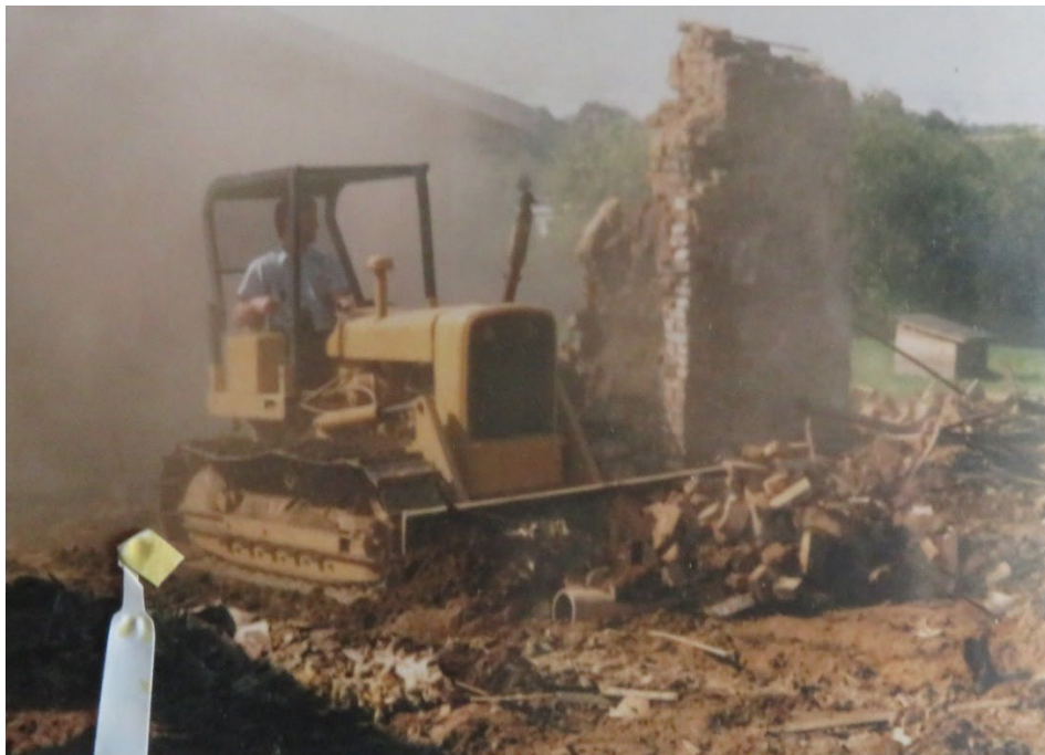
Fig. 11. A city worker removes debris from the back section of the house on High Street, which was completely demolished. The chimney and fireplace, which were centrally located between two rooms in that section, were obviously made of brick.
