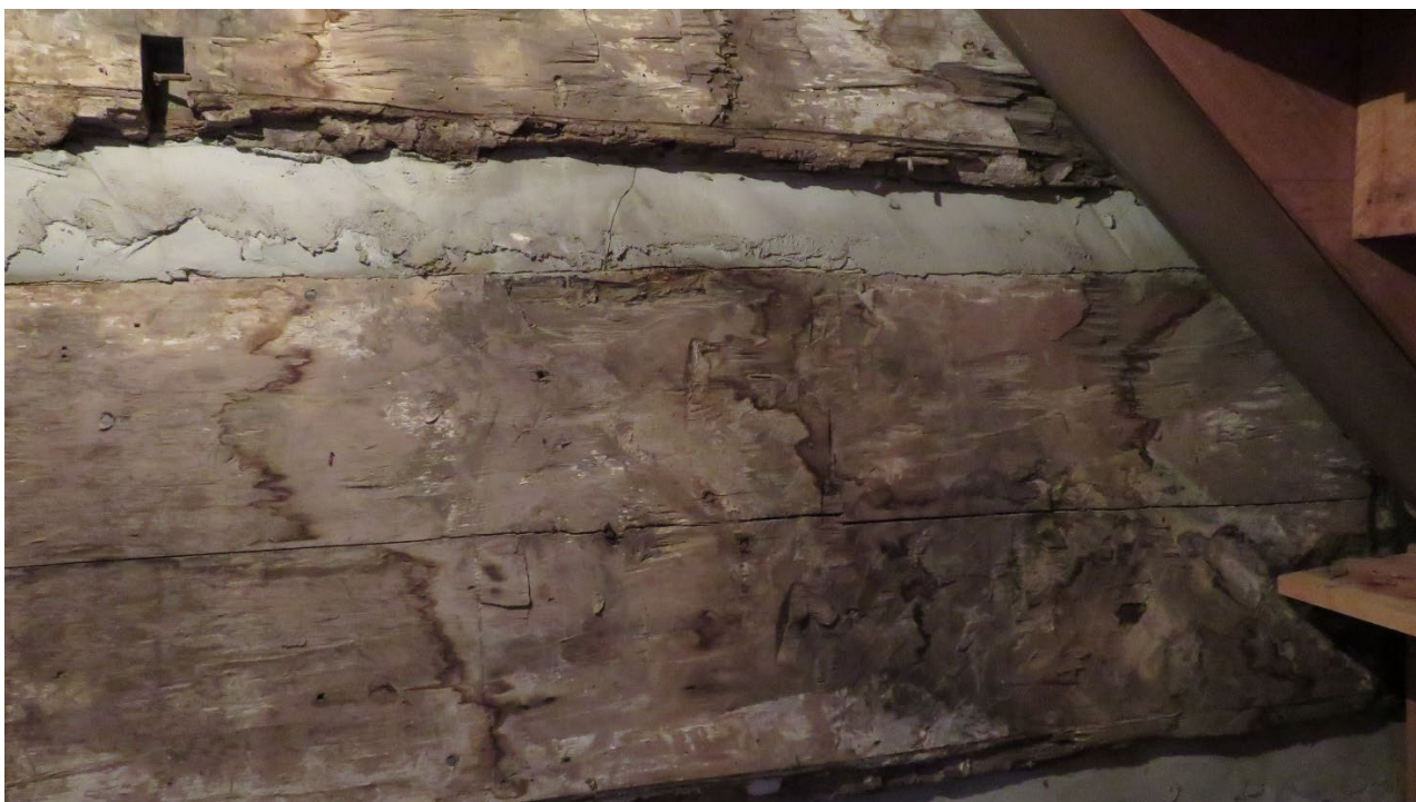
Fig. 9. Under the staircase, faint, but discernable, whitewash boundaries. a mortise, and nail holes indicate where the stairway was originally attached to the wall. It is positioned further from the front than the present staircase and is slightly less steep. Photo DRL
