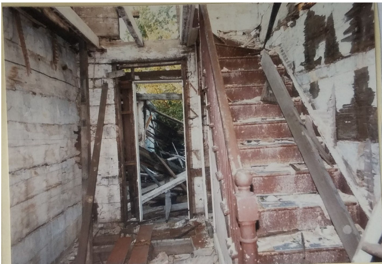
Fig. 8. This view shows several important features, such as the 90 degree spiral turn of the stairs at the top, as well as some excellent details of the Newell post. Another is the opening to the area under the stairs. The rough opening for the back door and the reduction framing is clearly visible. An example of the evidence that whitewash provides is shown above the stairs. The whitewash was probably applied as a finish to construction in 1848 or later, but before remodeling in 1853. When the walls were covered for the re-model, they were chipped where necessary to plumb the furring strips for the attachment of lath. So where the walls are bare, they were either covered when the whitewash was applied, or the whitewash was removed later, as in this case.
