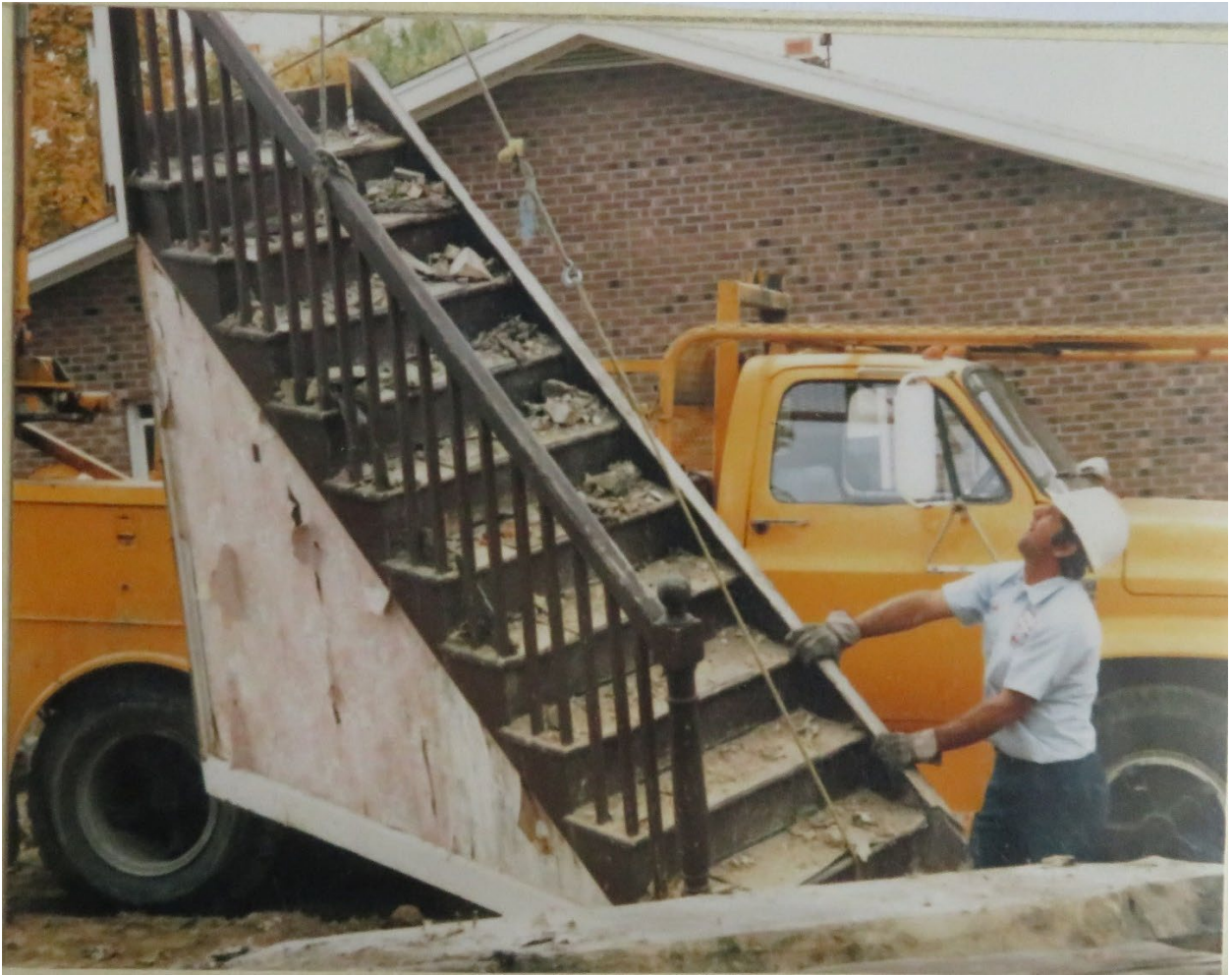
Fig. 5. This is the staircase as it was being removed with a crane. With hardwood steps, a railing, balusters, and turned Newell posts, it was much more modern than the rough-sawn pine which was put in its place.
