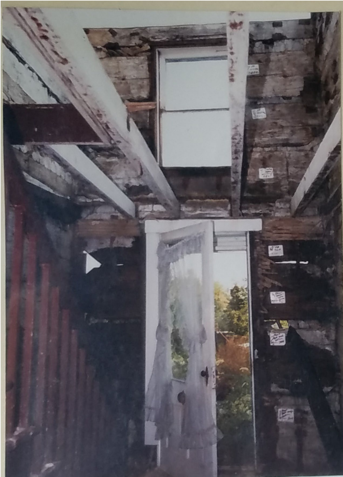
Fig. 7. The stairwell header frame is shown attached to the ceiling joists on the left. An existing mortise in the joists today marks the location.
