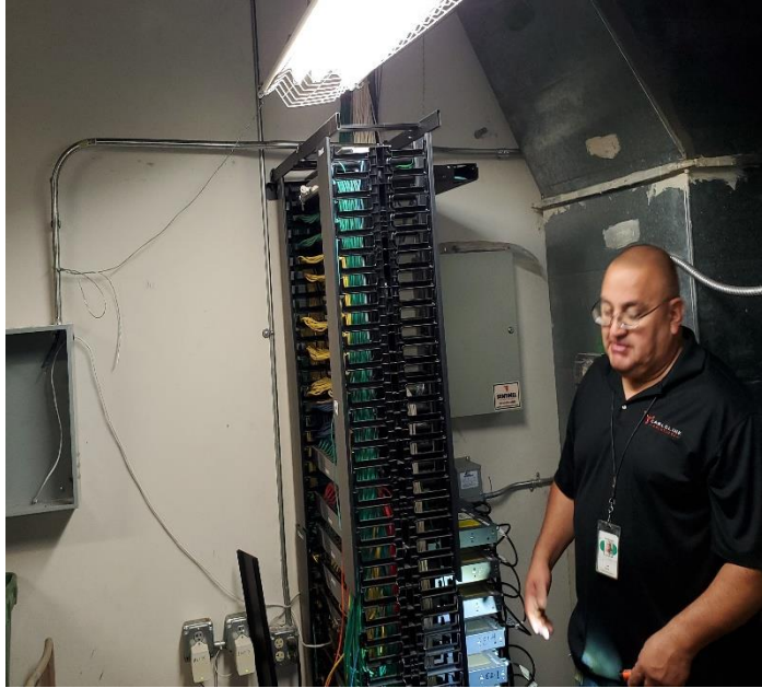
Lee Solis owner of Cablelink -Texas going over the plan for the work required for IDF E.
