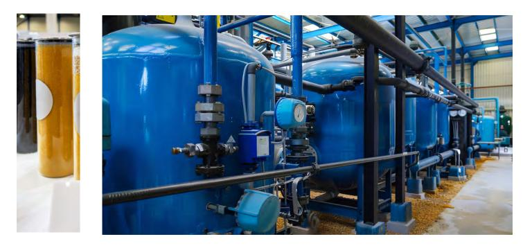
There are pre-formulated resin mixtures offered in various stoichiometric proportions to facilitate the production of ultrapure water (UPW). Common applications include stator cooling, Semiconductor,\* Pharma, labortaory, medical and RO permeate polishing.
