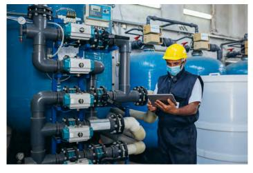
In multistage cation removal systems, Weak Acid Cation exchange (WAC) resins are utilized along with other components to effectively remove divalent ions.
