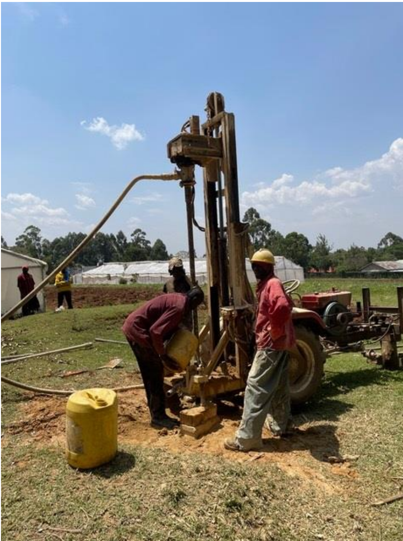
Borehole drilling with greenhouse in background
