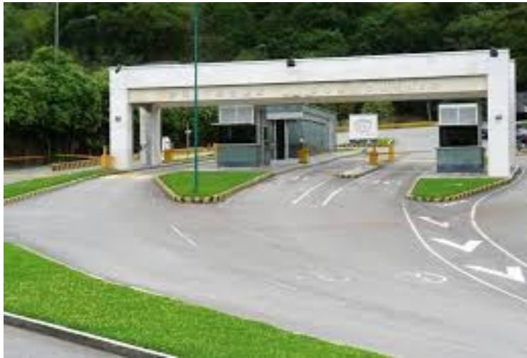
Porteria Principal Autopista Floridabca-Pcsta
