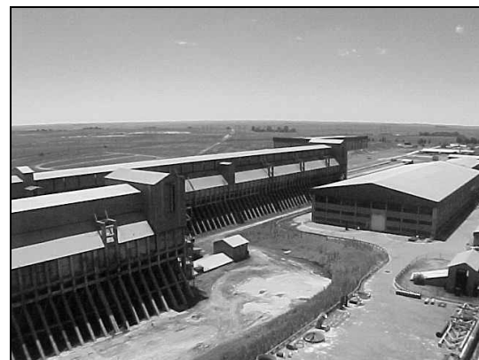
Fig 4: Coal feed into staiths on the left and the opposite side of the buildings, on the right. Photos taken from different angles, in reality the buildings have a straight linear shape
