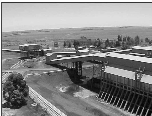
Fig 4: Coal feed into staiths on the left and the opposite side of the buildings, on the right. Photos taken from different angles, in reality the buildings have a straight linear shape
