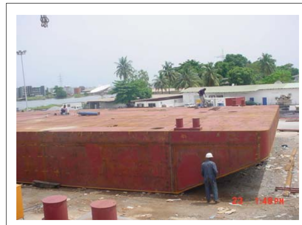
Prefabrication and erection of Barges JELUIS BERGER LAGOS
