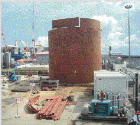
CONSTRUCTION OF 8500BBL STORAGE TANK- HALLIBURTON- ONNE PORT
