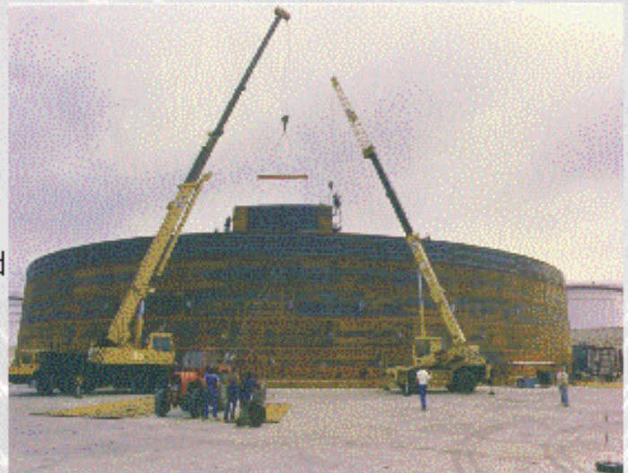
CONSTRUCTION OF 3 X 5M LITER TANKS ELF 1990
