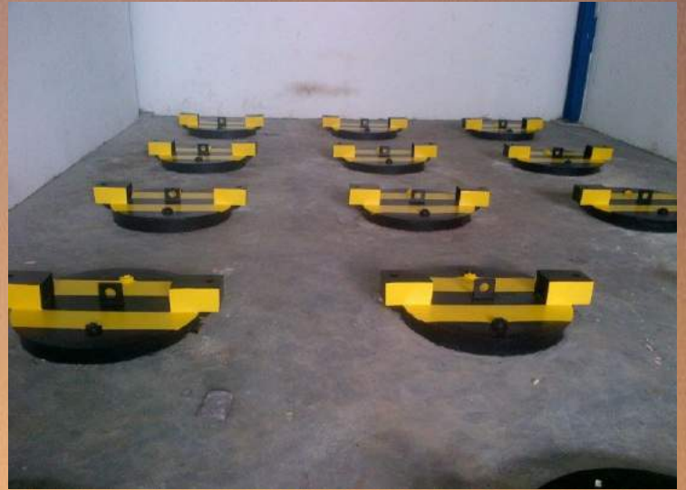
SCHLUMBERGER - D&M Underground Radioactive Source Storage Pit
