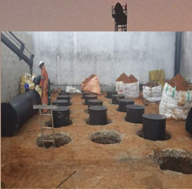
SCHLUMBERGER - D&M Underground Radioactive Source Storage Pit
