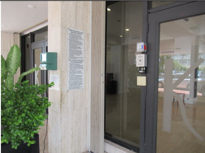
Common entry doors and shutters
