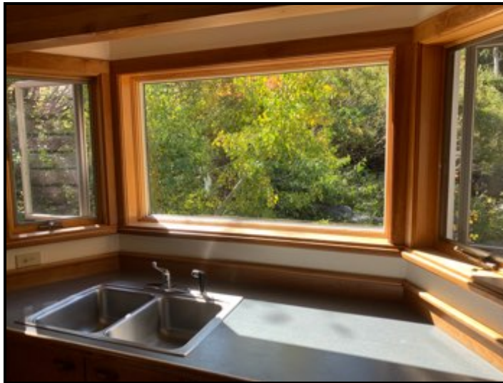
Operated windows appeared functional, at time of inspection.
