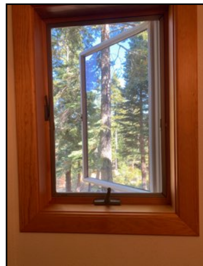
All were functional at the time of inspection.
