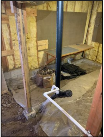
Appears Functional at time of inspection.
