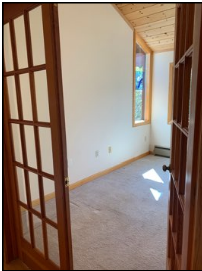
Satisfactory at time of inspection. No concerns.
