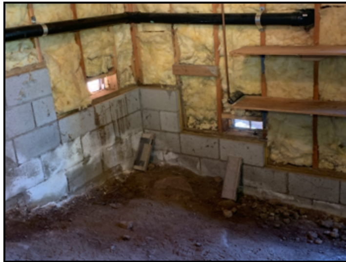
Adequate ventilation observed.
