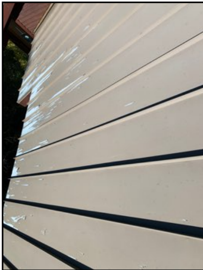
Paint on metal roof starting to fade or areas of exposed metal. Recommend contacting licensed roofer for further guidance and repairs.
