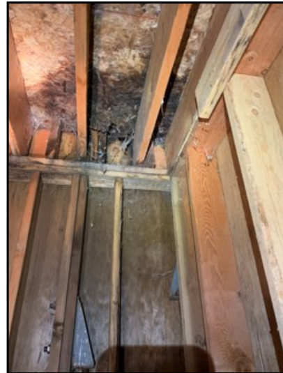
Evidence of moisture staining or wood rot observed on subfloor. Recommend contacting licensed professional for further evaluation and repairs.
