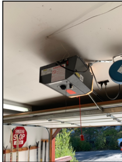
Chain drive opener noted.
