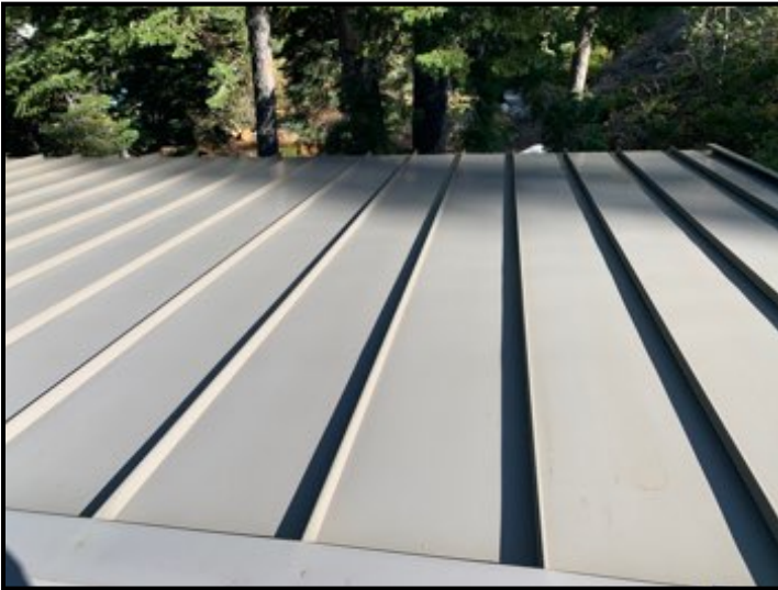
Most areas satisfactory at time of inspection except where otherwise noted
