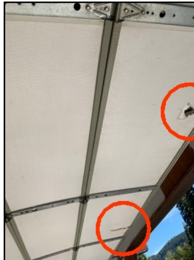
Damage to garage door insulation observed.
