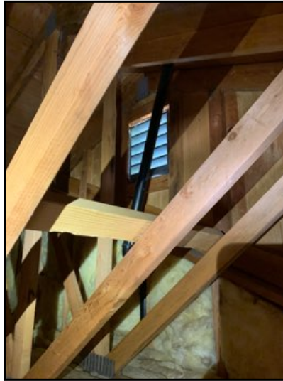
ABS plumbing vents
