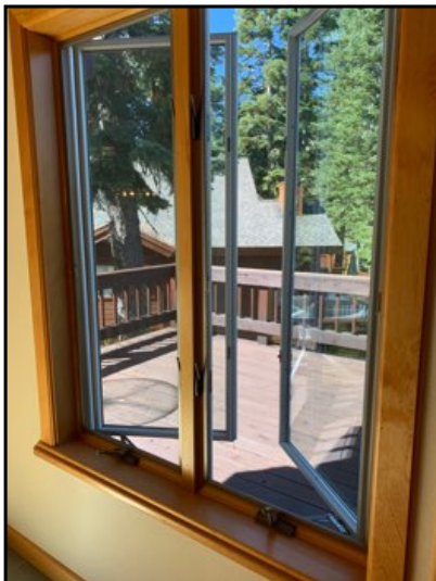
Operated windows appeared functional, at time of inspection
