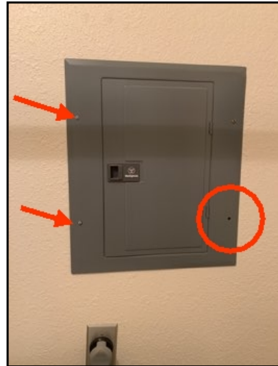
Incorrect screws on laundry panel. Recommend replacing with correct screws
