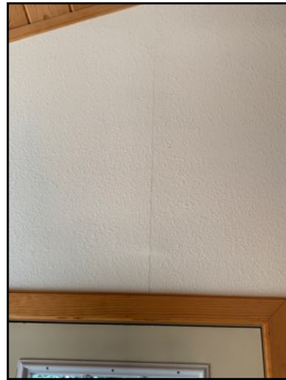
Small cracking in the wall finish is noted. Commonly caused by the joint compound (spackle) drying too quickly during application, or by expansion and contraction during snow loads.
