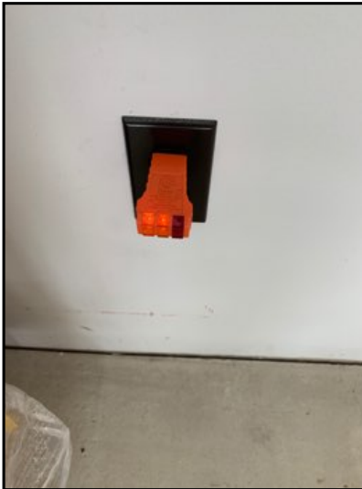
All appear operational at time of inspection.
