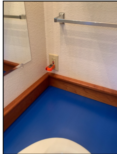
GFCI in place and operational
