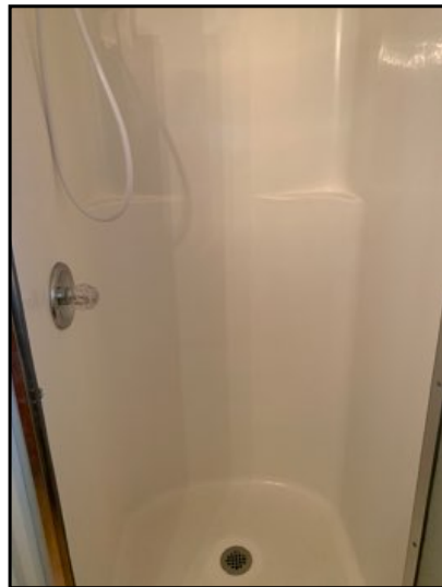
Fiberglass surround noted.
