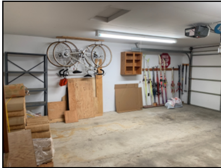
Appeared satisfactory, at time of inspection.
