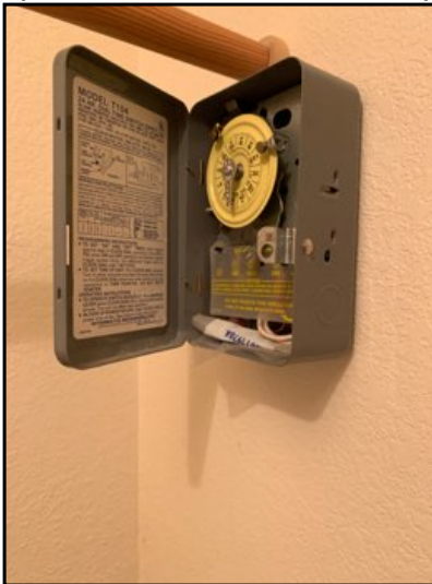
Timer for instant hot water observed. Instant hot unit not located during inspection. Water was hot on demand at time of inspection.
