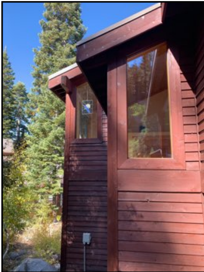
Components appeared in satisfactory condition at time of inspection.
