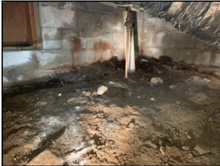
High moisture in soil observed in corner of structure.
