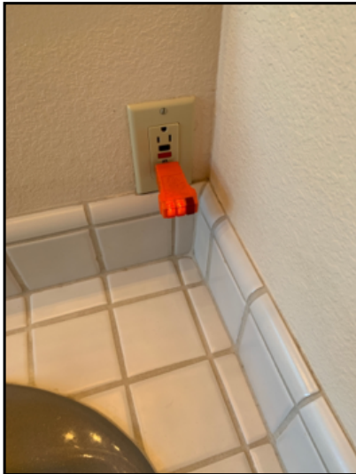
GFCI in place and operational
