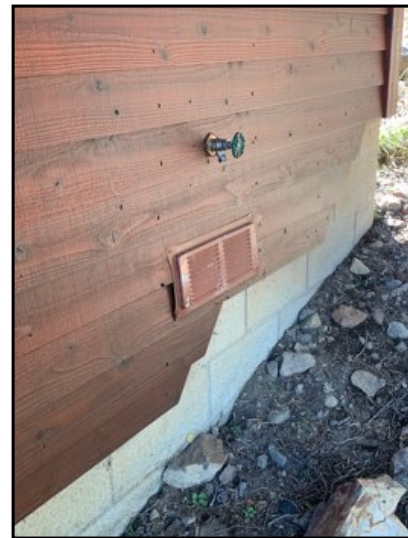
Not functional at one or more locations, further review and repair recommended.
