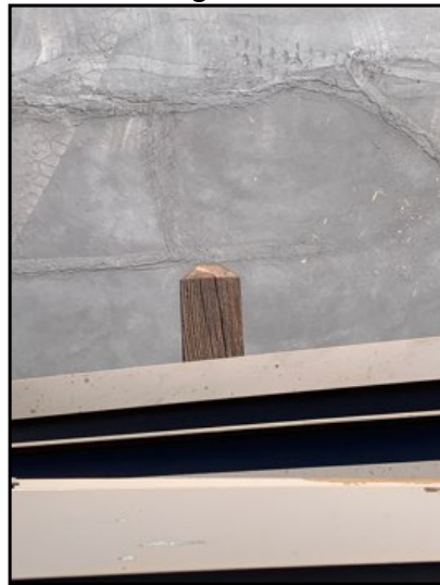
Recommend installation of beam caps to prevent wood rot or deterioration.
