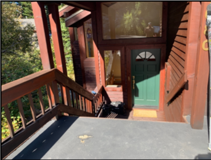
Handrail not graspable. By today's standards, rails should be configured so that a hand may grasp around a rail for safety.
