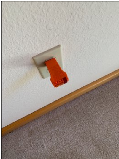
All appear operational at time of inspection.
