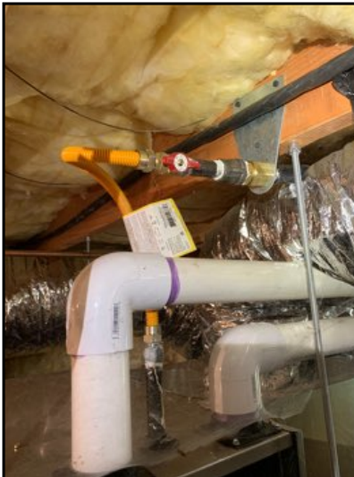
Gas shut off valves were present and functional.
