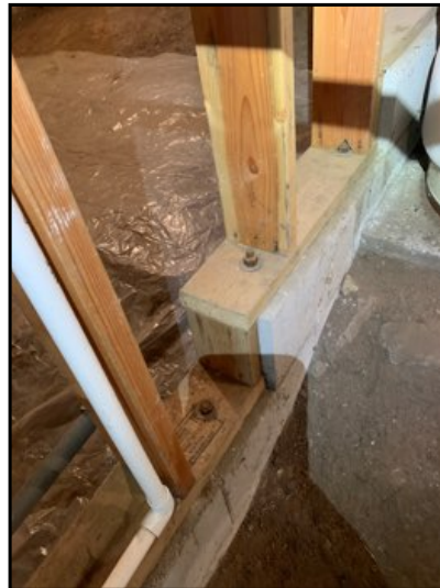
The anchor bolts were inspected and appear to be serviceable.
