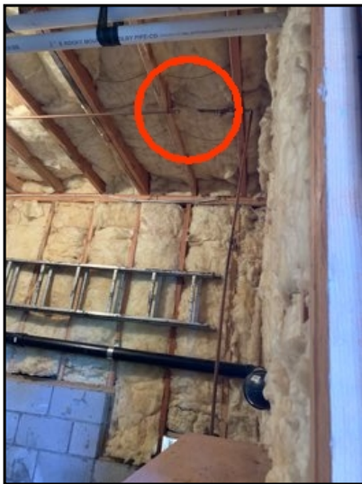
Water line to exterior faucet has been capped and no longer in service.
