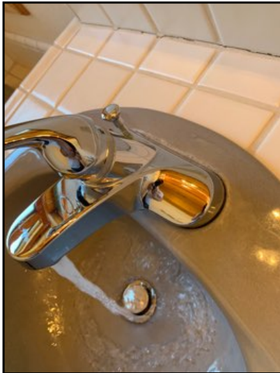
Pull stop not functional.
