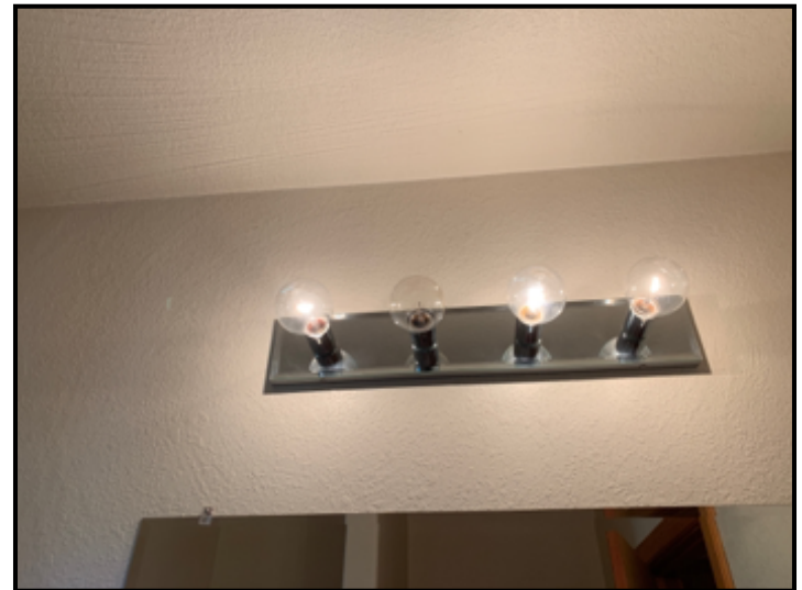
Light bulb out. Replace and recheck
