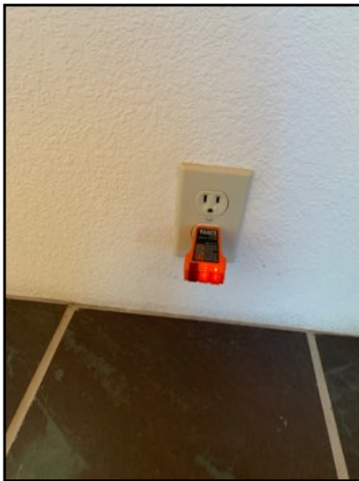
All appear operational at time of inspection.
