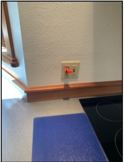
All appear operational at time of inspection.
