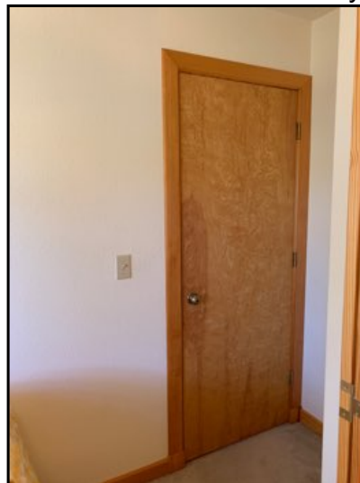
Satisfactory at time of inspection. No concerns.
