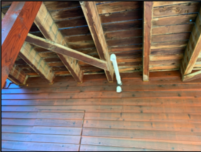
Lag bolts not present.
