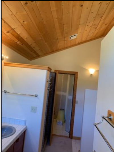
No concerns at time of inspection.
