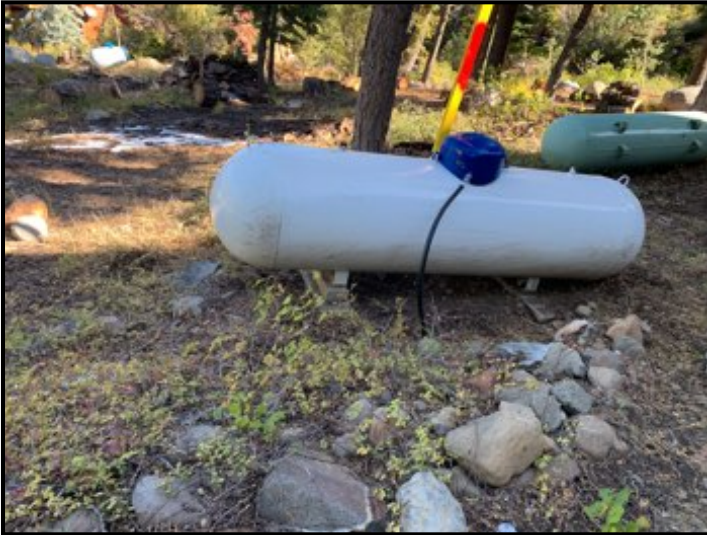
Propane tank is present. No odors detected. Shut off valve present and appeared functional at time of inspection.
