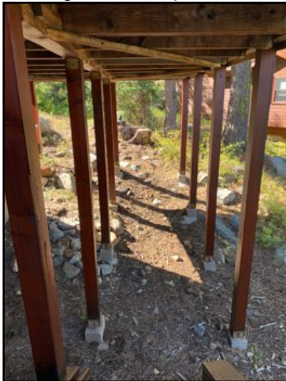
Appeared functional at time of inspection.
