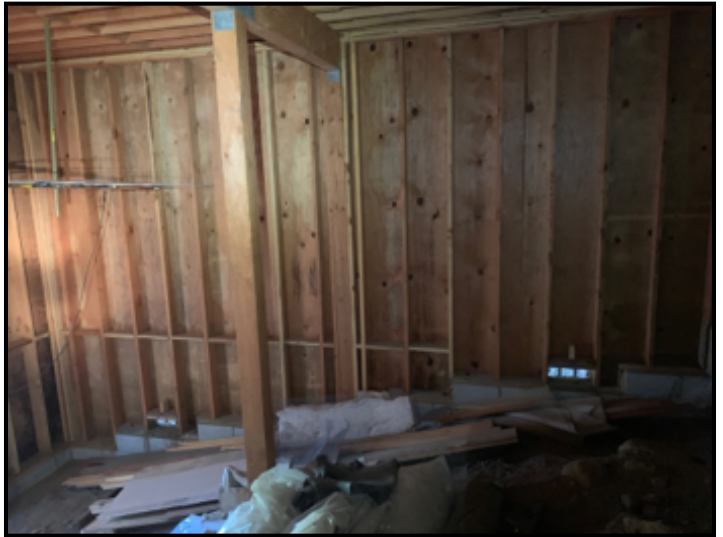
Satisfactory at time of inspection.
