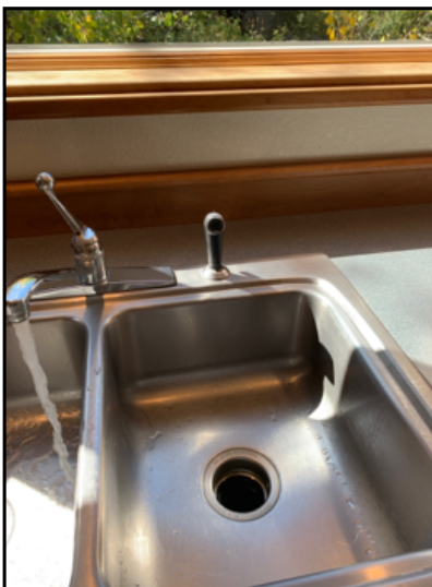
The spray wand was operated and was functional.
