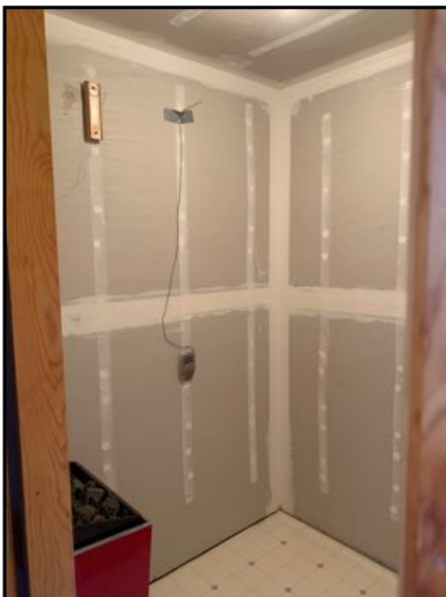
Unfinished sauna walls observed. Do not recommend using until finished. Testing of saunas are not within the scope of a home inspection.
