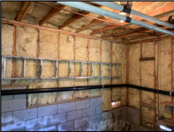
Satisfactory at time of inspection.
