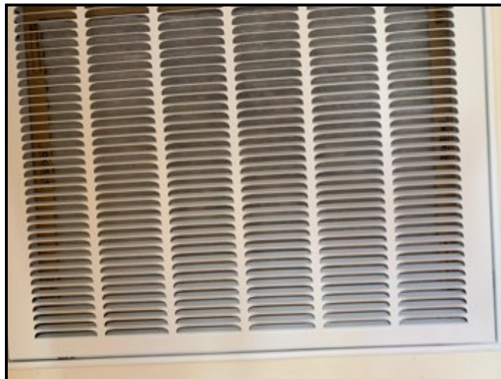
Satisfactory at time of inspection. No concerns.
