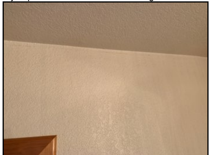
Small cracking in the wall finish is noted. Commonly caused by the joint compound (spackle) drying too quickly during application, or by expansion and contraction during snow loads.
