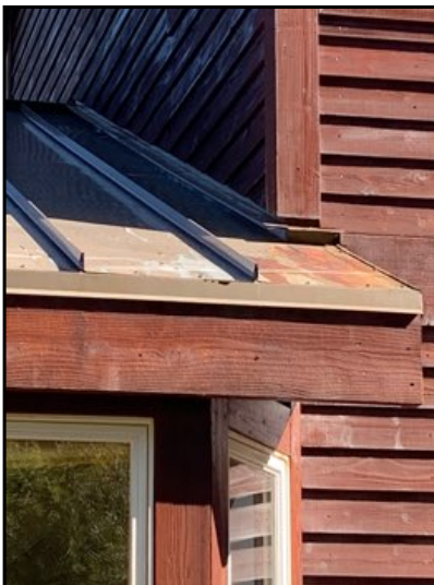
Surface rust observed. Recommend review by licensed professional for further guidance and repairs.
