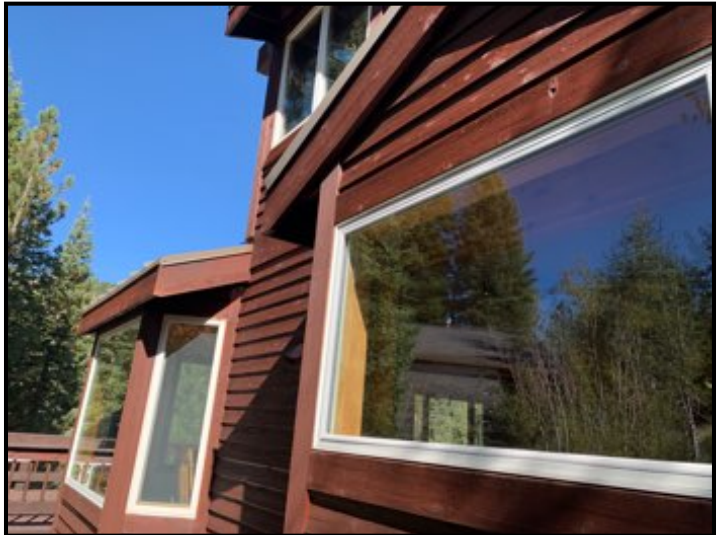
Components appeared in satisfactory condition at time of inspection.
