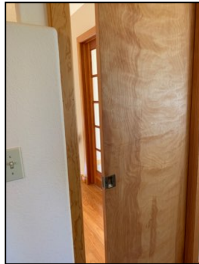
Satisfactory at time of inspection. No concerns.
