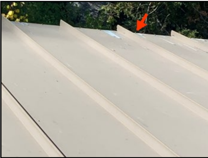
Screws are backing out. Recommend resetting and resealing.
