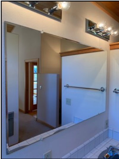
No deficiencies noted at time of inspection.
