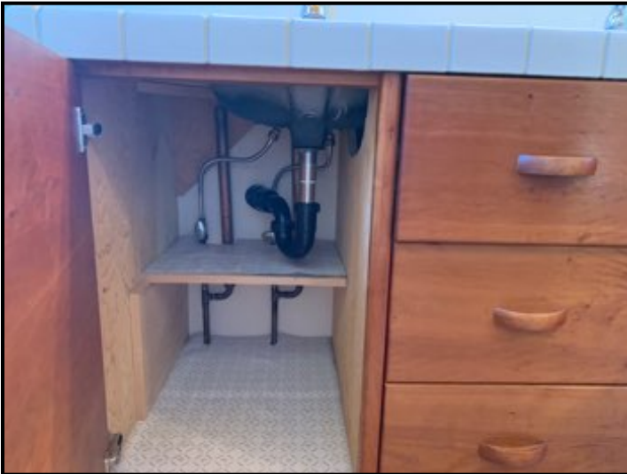
No deficiencies noted at the time of inspection.
