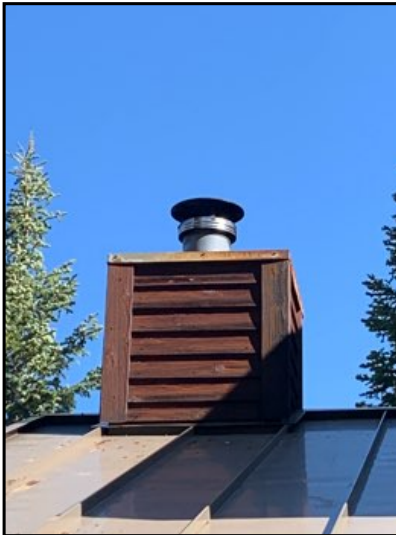
Rain cap and spark arrester satisfactory at time of inspection.
