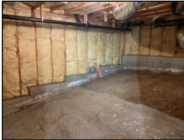
Efflorescence observed; this is a mineral deposit left behind from exterior water infiltration.
