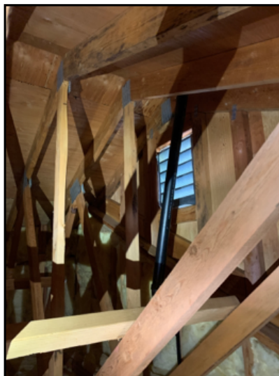
Gable louver vents noted.
