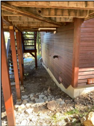
Most areas satisfactory at time of inspection except where otherwise noted.
