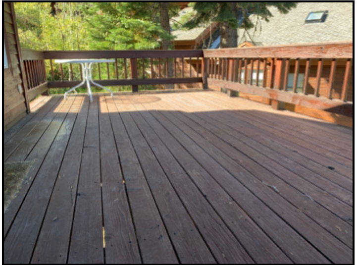
Appeared functional at time of inspection.
