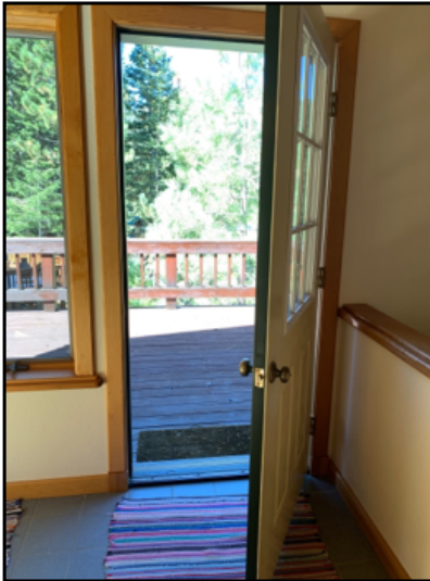
The hinged patio door was functional during the inspection.
