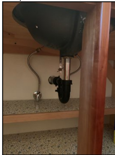
No deficiencies noted at the time of inspection.
