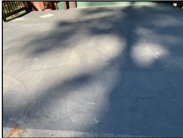
Driveway in good shape for age and wear. No deficiencies noted.
