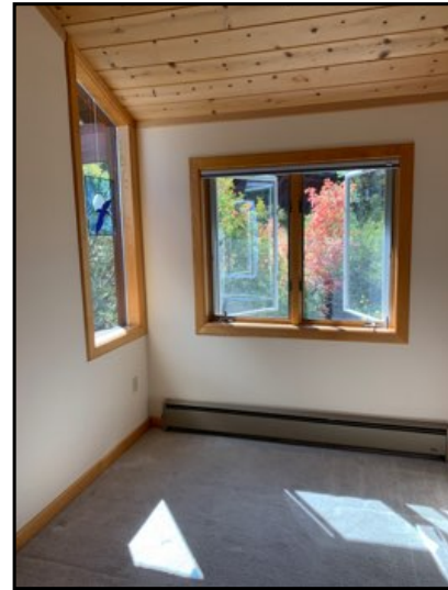
Operated windows appeared functional, at time of inspection.
