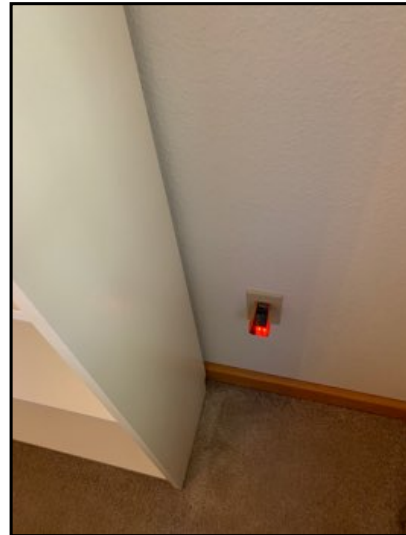
All appear operational at time of inspection.
