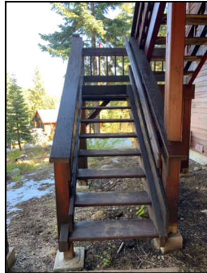
Handrail not graspable. By today's standards, rails should be configured so that a hand may grasp around a rail for safety.
