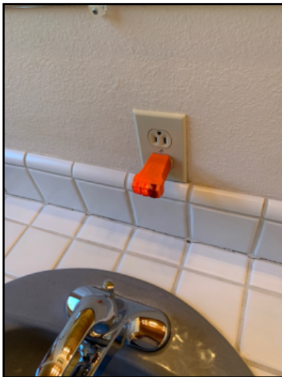
All appear operational at time of inspection.
