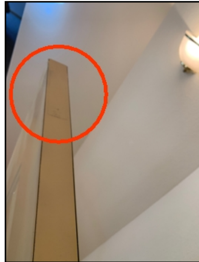
Fire rating stamp has been painted over. Door is most likely fire rated, however unable to determine fire rating at time of inspection.
