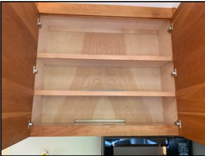
Appeared functional and in satisfactory condition, at time of inspection.
