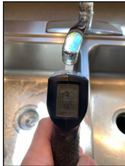
Hot water temperature above 120 degrees F. Recommend adjustment of water heater to prevent scalding.
