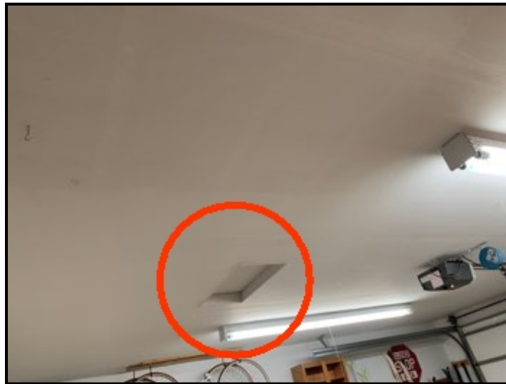
Hole in the ceiling is a breach in the fire protection.
