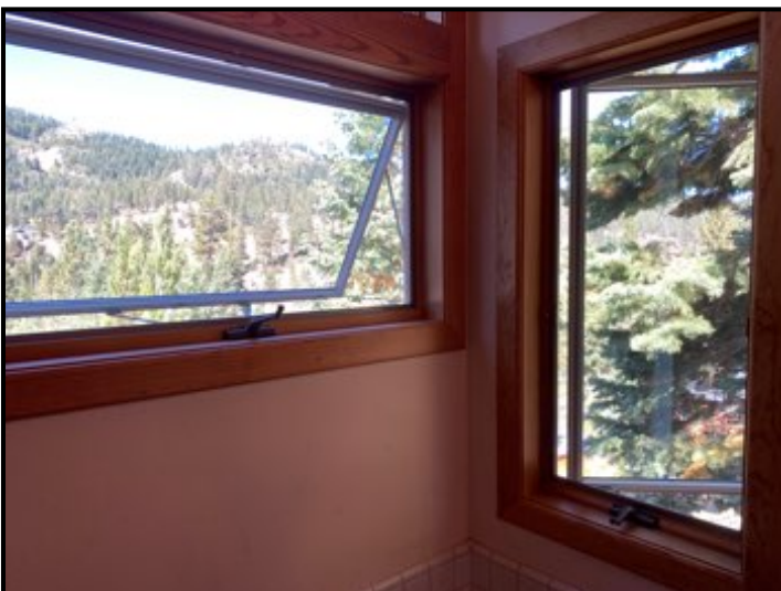
All were functional at the time of inspection.
