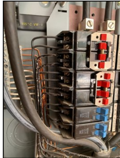
All of the circuit breakers appeared serviceable.
