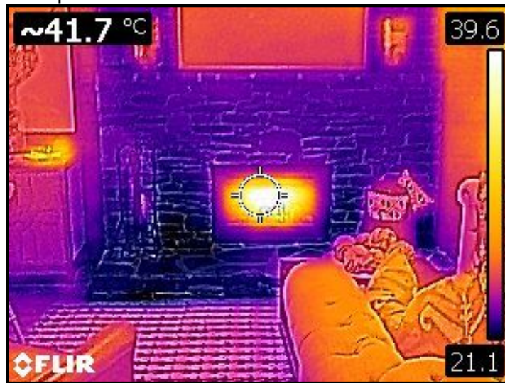
Gas fireplace operational at time of inspection.
