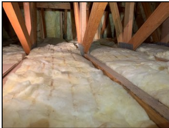
Insulation appears adequate.
