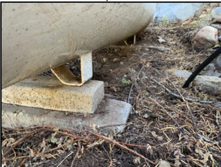
Recommend securing propane tank to base
