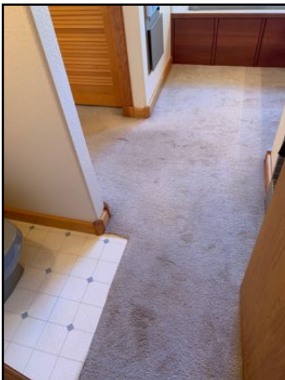
No deficiencies noted at time of inspection
