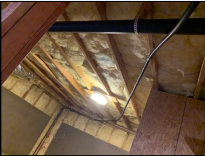
Not completely visible to inspect due to being covered by insulation.
