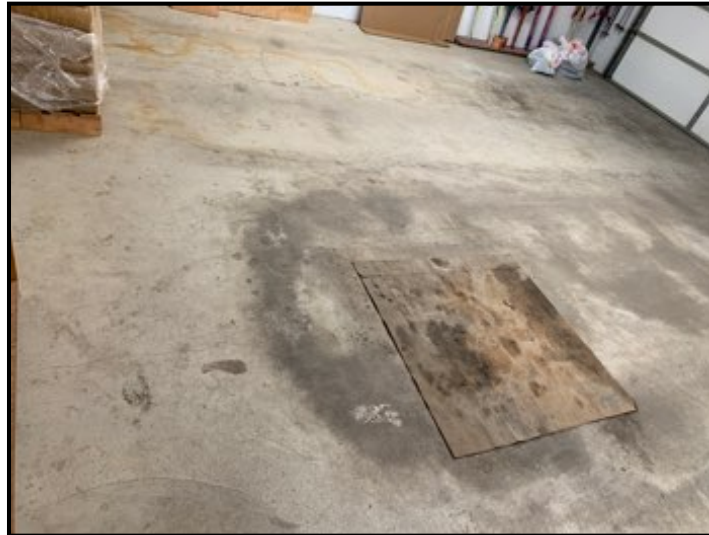
Satisfactory at time of inspection. No safety or functional concerns.
