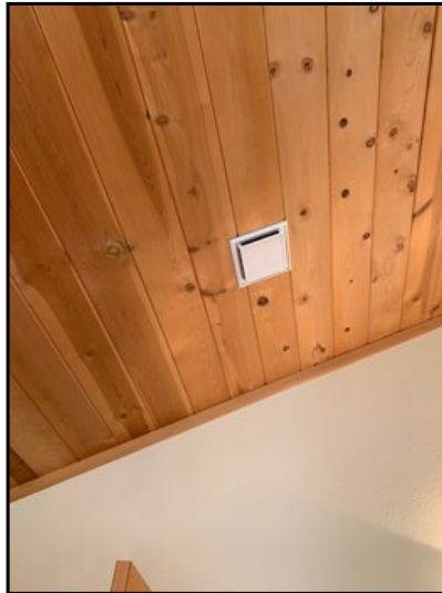
The bath fan was operated and no issues were found.
