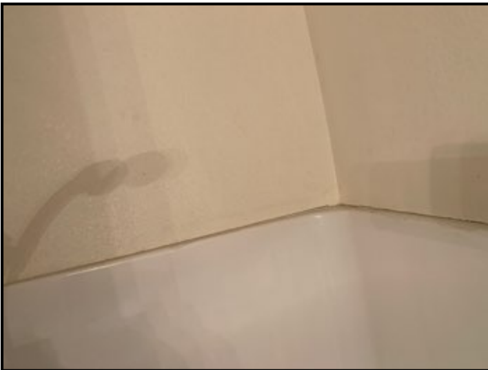
Recommend caulking as required.
