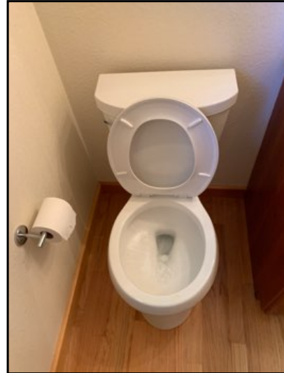
Observed as functional and in good visual condition.
