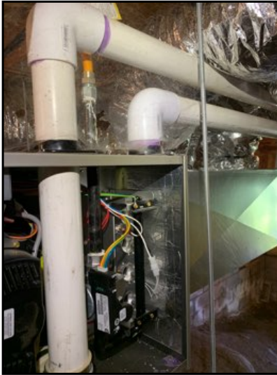
All appeared functional at the time of inspection.
