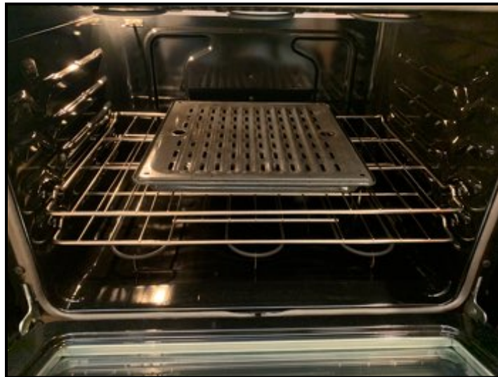
All heating elements operated when tested.
