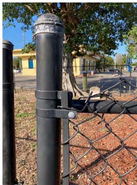
02.10.25 The fence and gate were damaged at the historical cemetery. It appears a vehicle backed into the fence.
