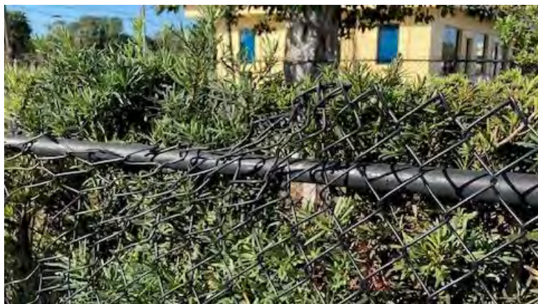
02.10.25 The fence and gate were damaged at the historical cemetery. It appears a vehicle backed into the fence.
