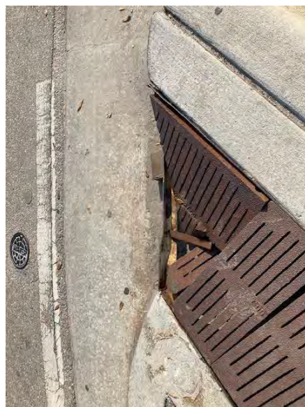
2.10.25 Damaged grates were reported to Webber, FDOT's Subcontractor, for repair at S 4 th St and S 2 nd St
