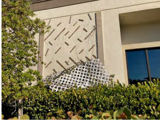
Lattice work failure on storefront
