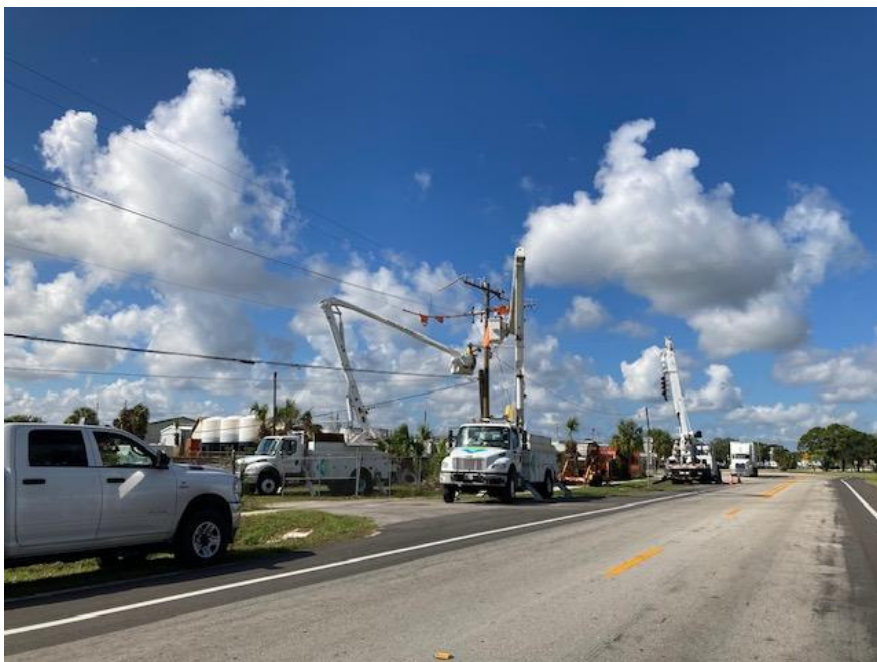
10.21.25 New wire installation along CR 846 E, just west of Airpark Blvd
