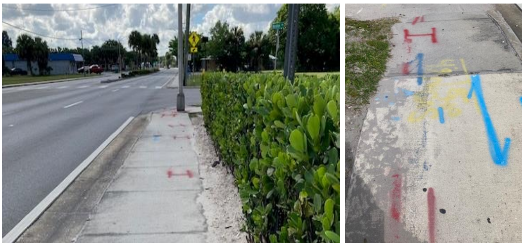
10.21.24 KCA's Surveyor, T2, completing the SUEs and surveying for the First Street PH2 Project
