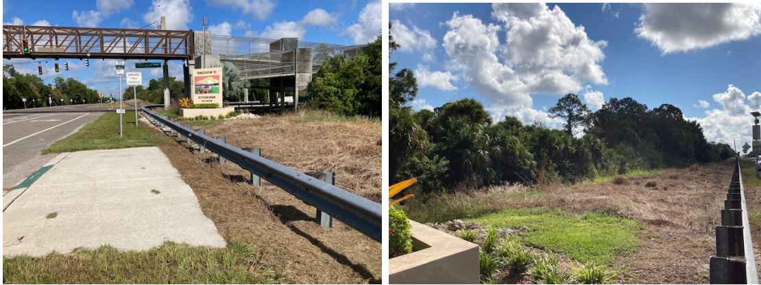
12.21.25 FDOT's Subcontractor, Webber, is keeping the brush mowed for clear sightlines to the Panther Welcome Sign
