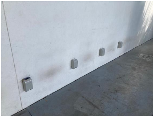
10.21.25 Simmonds Electrical put covers on the bandshell and trellis electrical outlets with an new electrical panel to turn power on-off
