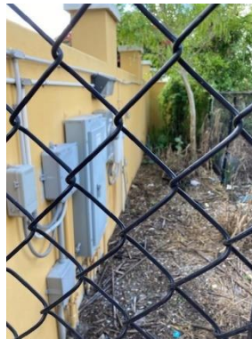
10.21.25 Simmonds Electrical put covers on the bandshell and trellis electrical outlets with an new electrical panel to turn power on-off
