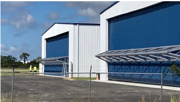
10.21.25 Construction completed on the new hangers
