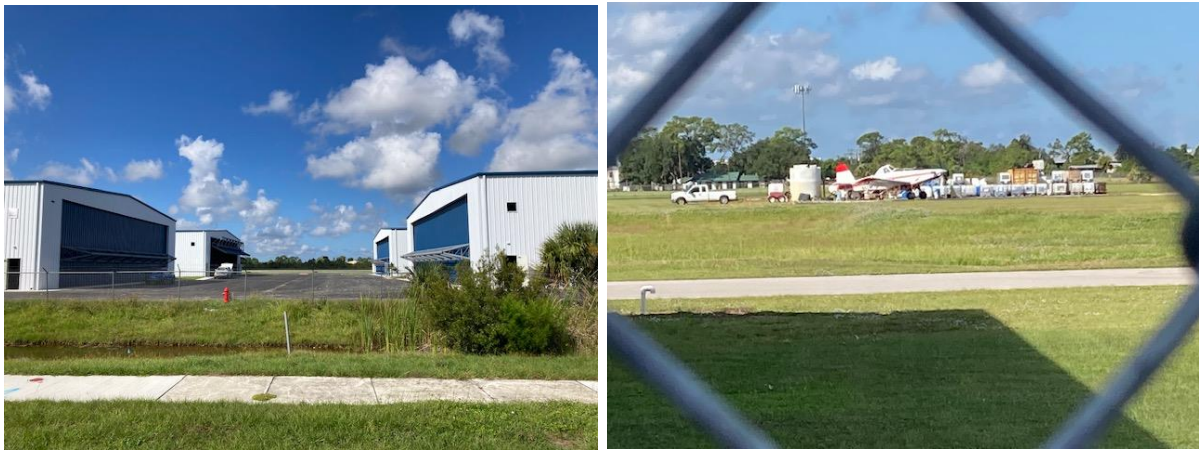
10.21.25 New hangers at Immokalee Airport are completed
