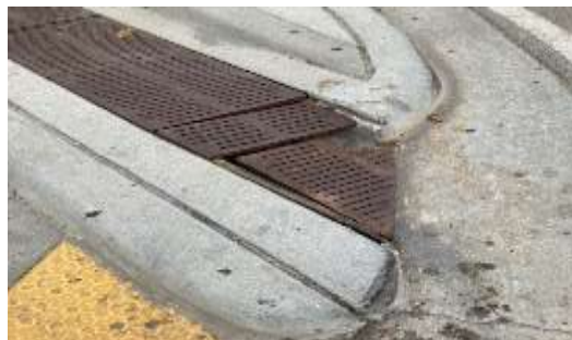
03.10.25 Sidewalk grate in front of Mr. Taco to be replaced by A&M and damaged grate at S 2 nd Street to be repaired by FDOT/WWebber
