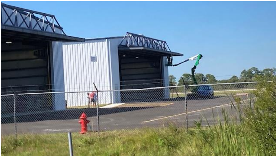
11/3/25 Improvements continue to be made to the airport hangers and grounds.
