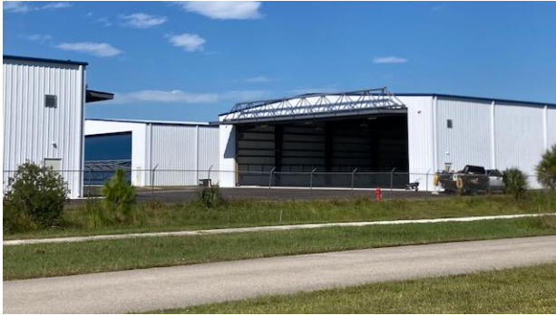
11.3.25 Construction completed on the new hangers
